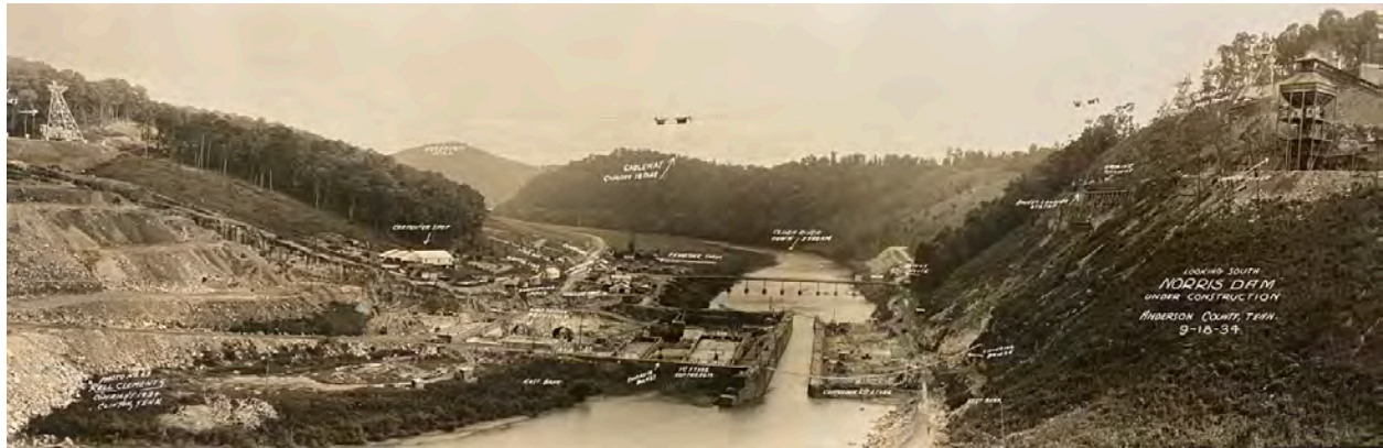
The construction site along the Clinch River, 1934.
