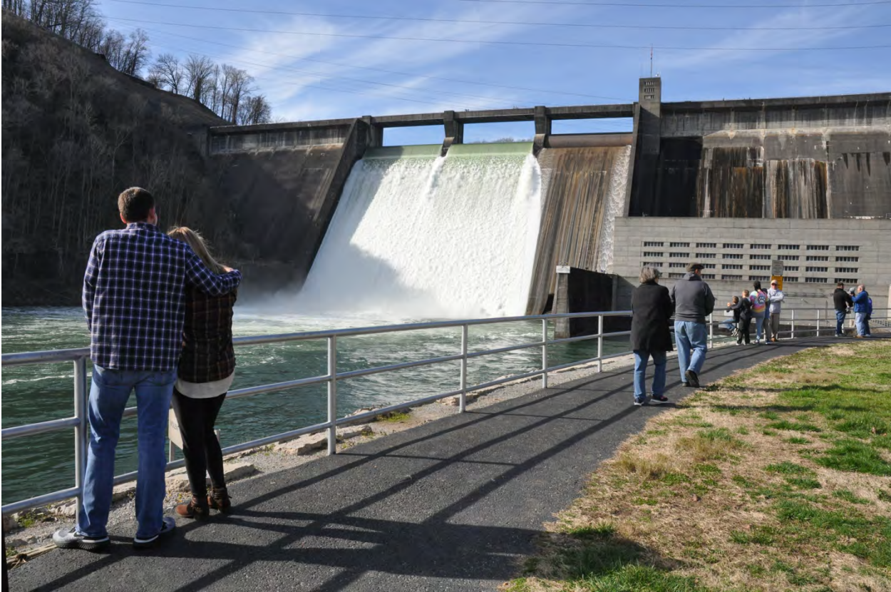
This view of the face of the dam and the release of the lake water, turn off Norris Freeway onto Powerhouse Way.
