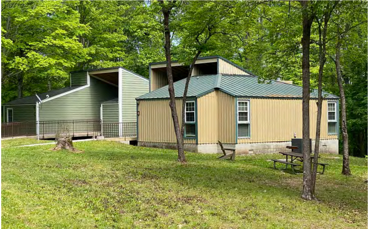
Two of the rental cabins in the west side of Norris Dam State Park.
