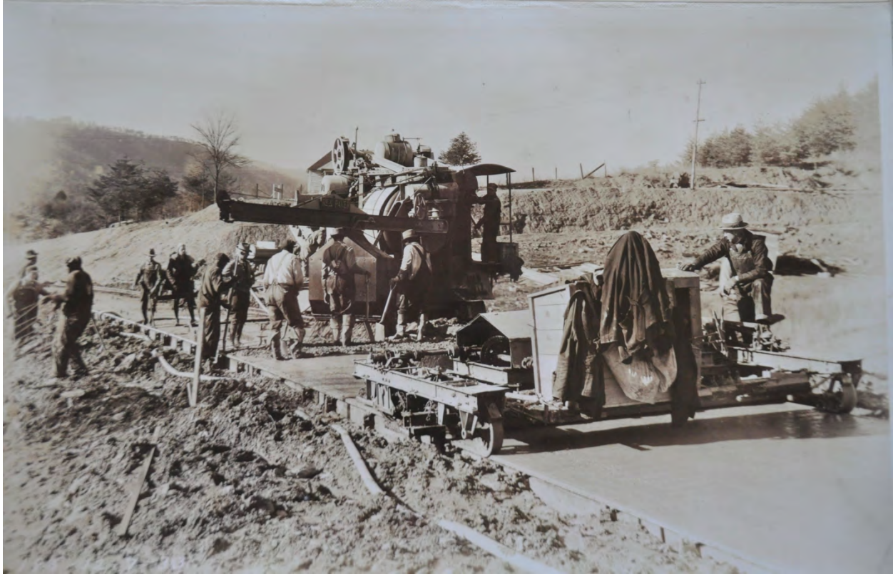
The TVA construction crew laying the concrete for the Freeway in 1934.
