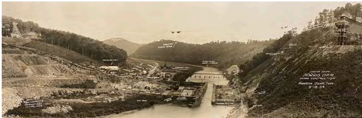
The Norris Dam construction on the Clinch River in 1934.
