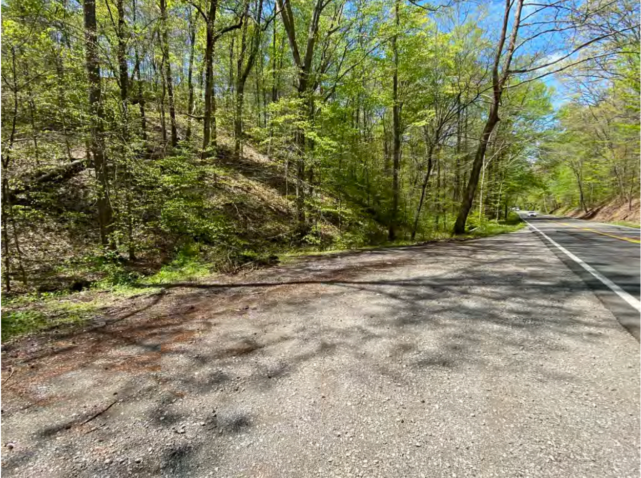
One of the pull-offs along the Freeway.
