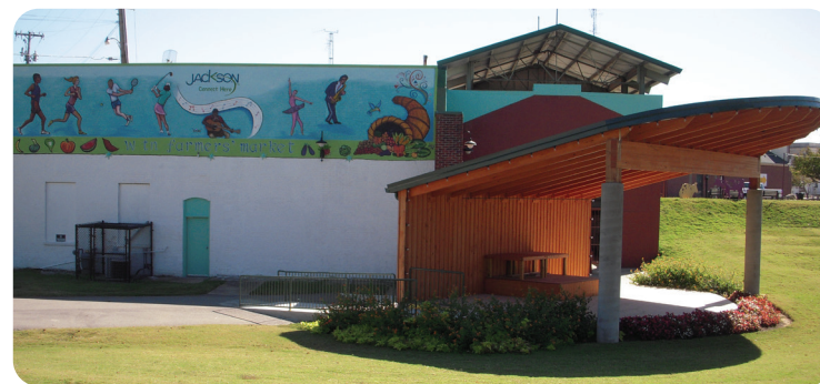
The completed brownfield site cleanup turned the property into an urban pocket park and outdoor amphitheater that complements the vision of downtown Jackson's revitalization, and a new 20-acre development, the Jackson Walk community, grew around the former Citizens Gas and Light Property.
