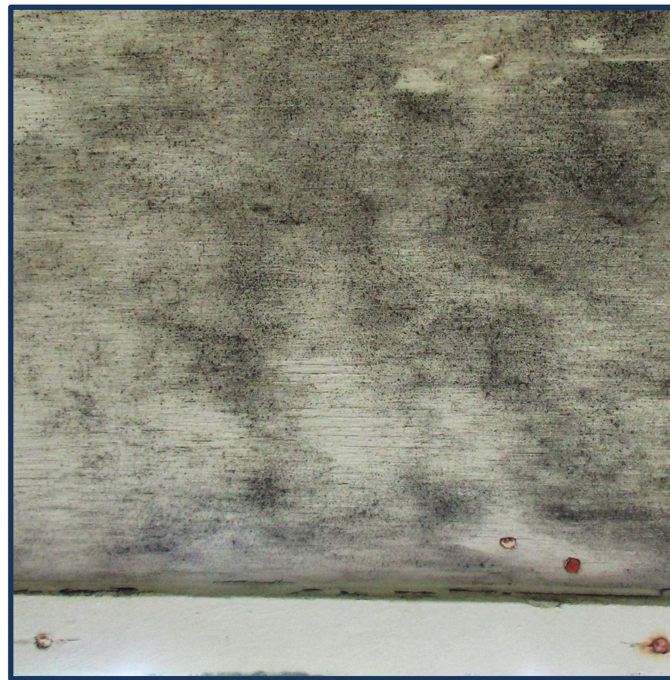
Too much moisture allows mold to grow. Molds are allergens and can be asthma triggers.
