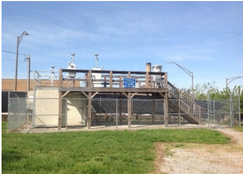
Figure 3.1 Air Lab Site Photo
