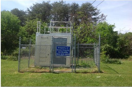
Figure 3.16 East Knox Site Photo
