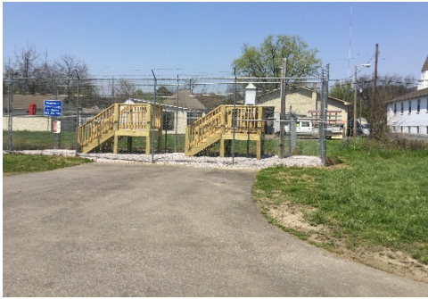
Figure 3.6 Ameristeel Site Photo
