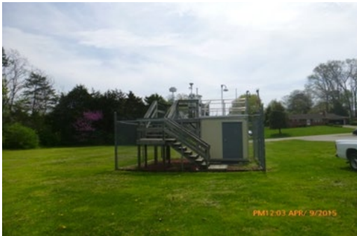
Figure 3.26 Springhill Site Photo
