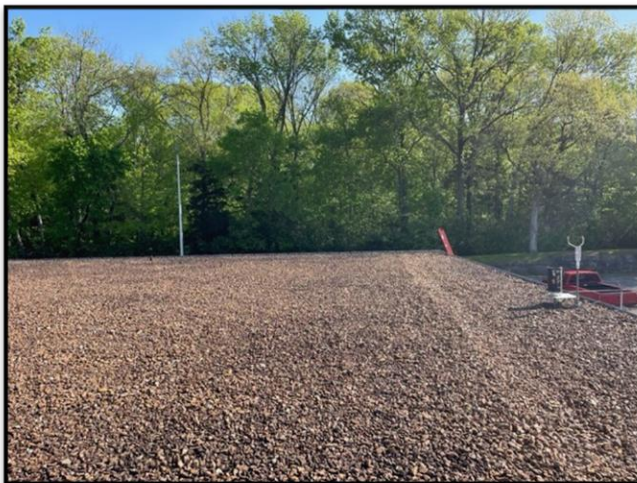
Figure 3-9: Percy Priest Dam (EAST)
