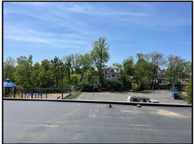
Figure 3-11: Lockeland Elementary (SOUTH)
