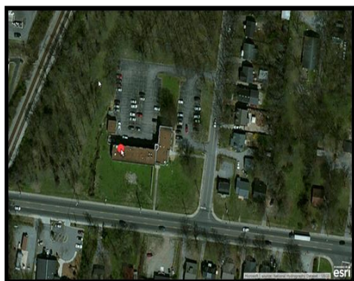
Figure 2-2: East Health Center (Aerial View)
