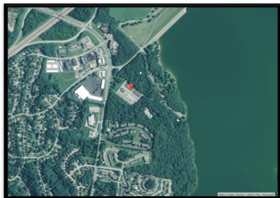
Figure 2-4: Percy Priest Dam Site (Aerial View)
