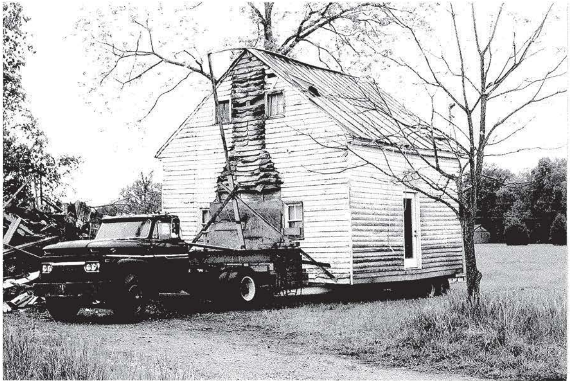
Figure 5. Adams Inn building being moved from site.
