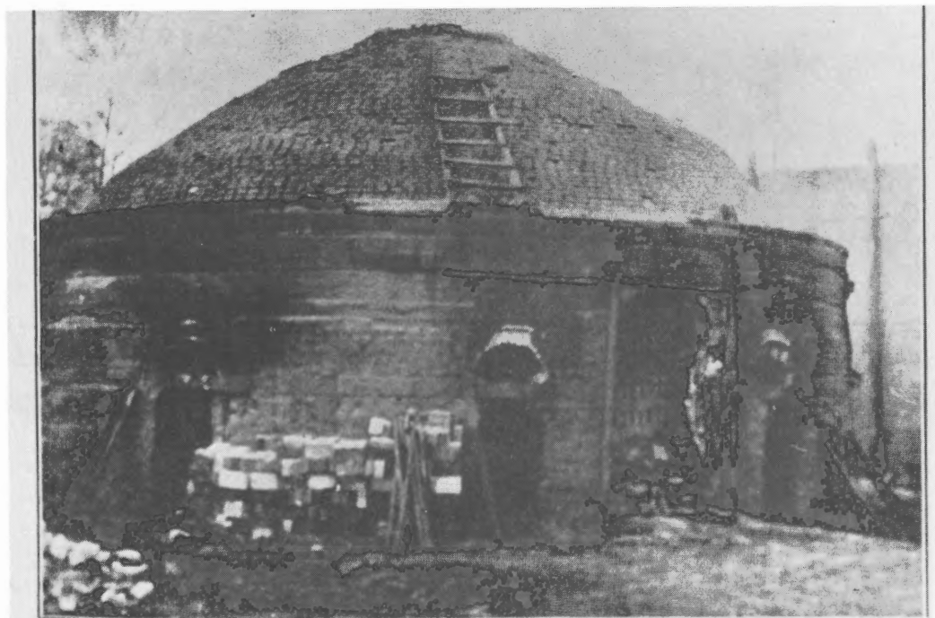
FIG. B. TYPICAL DOWNDRAFT BEEHIVE KILN, SHOWING FINISHED BURN. SOUTHERN TILE AND BRICK WORKS, GILMORE, TENNESSEE.
