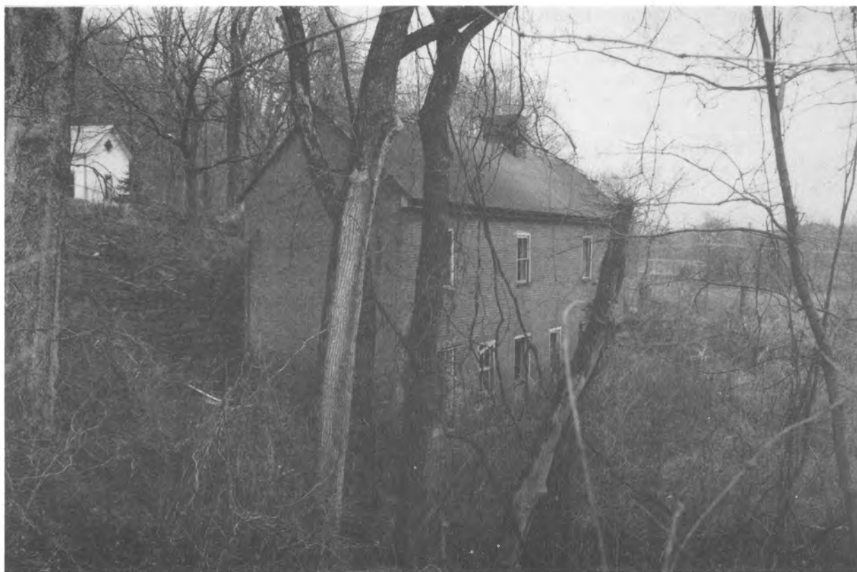
Figure 34. Cumberland Furnace Company Store (Dickson County 328).
