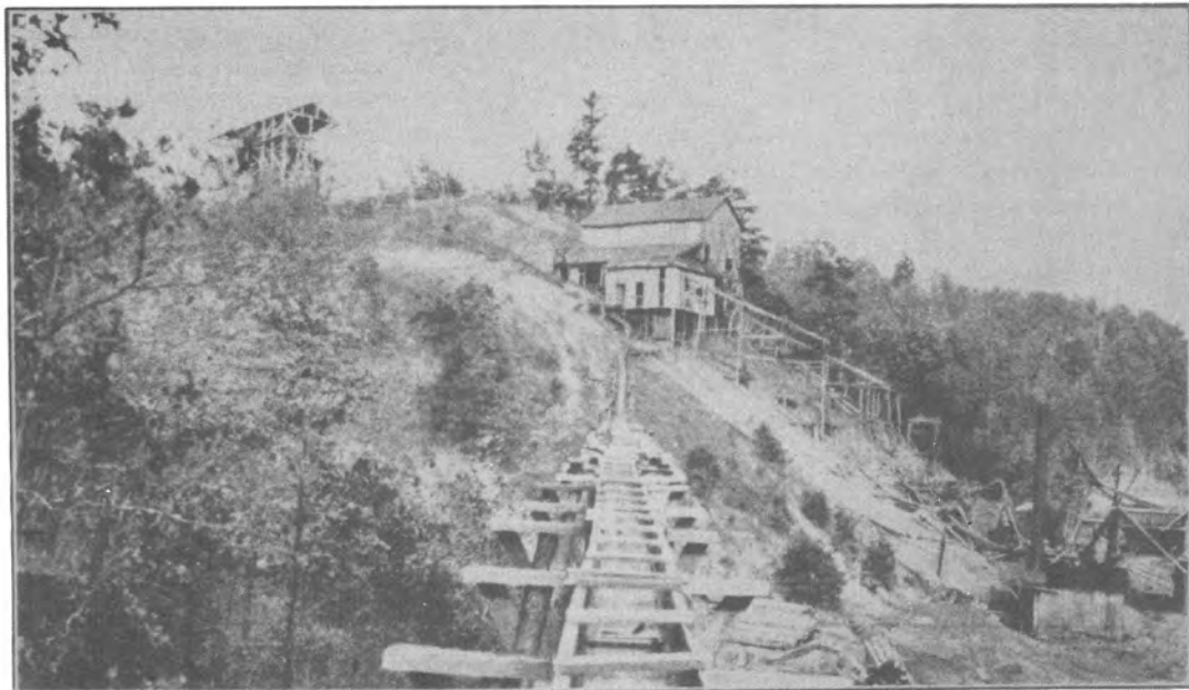
(B) Tipple, ore washer, ore bin, and waste flume at Aetna brown iron ore mine of former Bon Air Coal & Iron Corporation, 1921.
