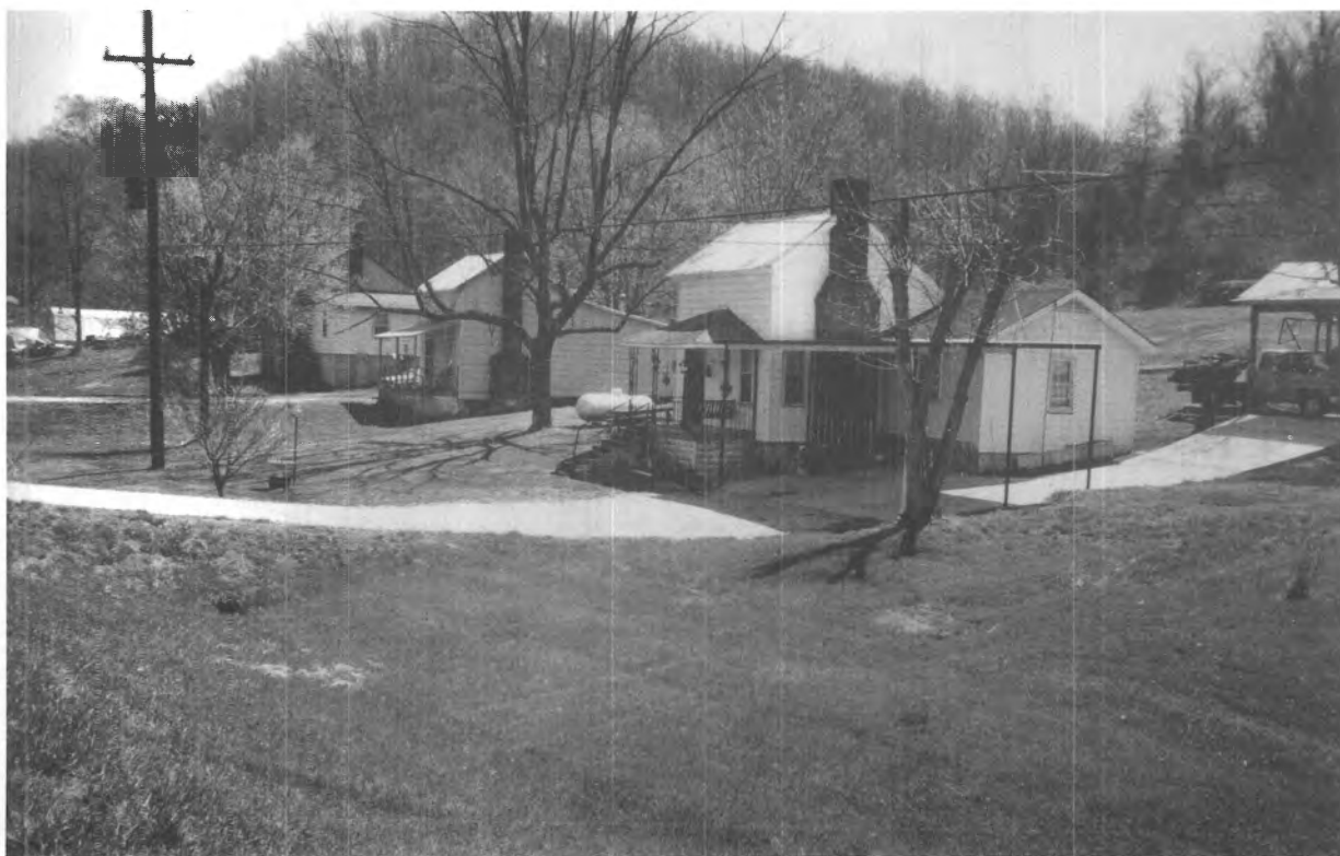
Figure 44. Rockdale House Number 1 (Maury County 423, with 424 to left).
