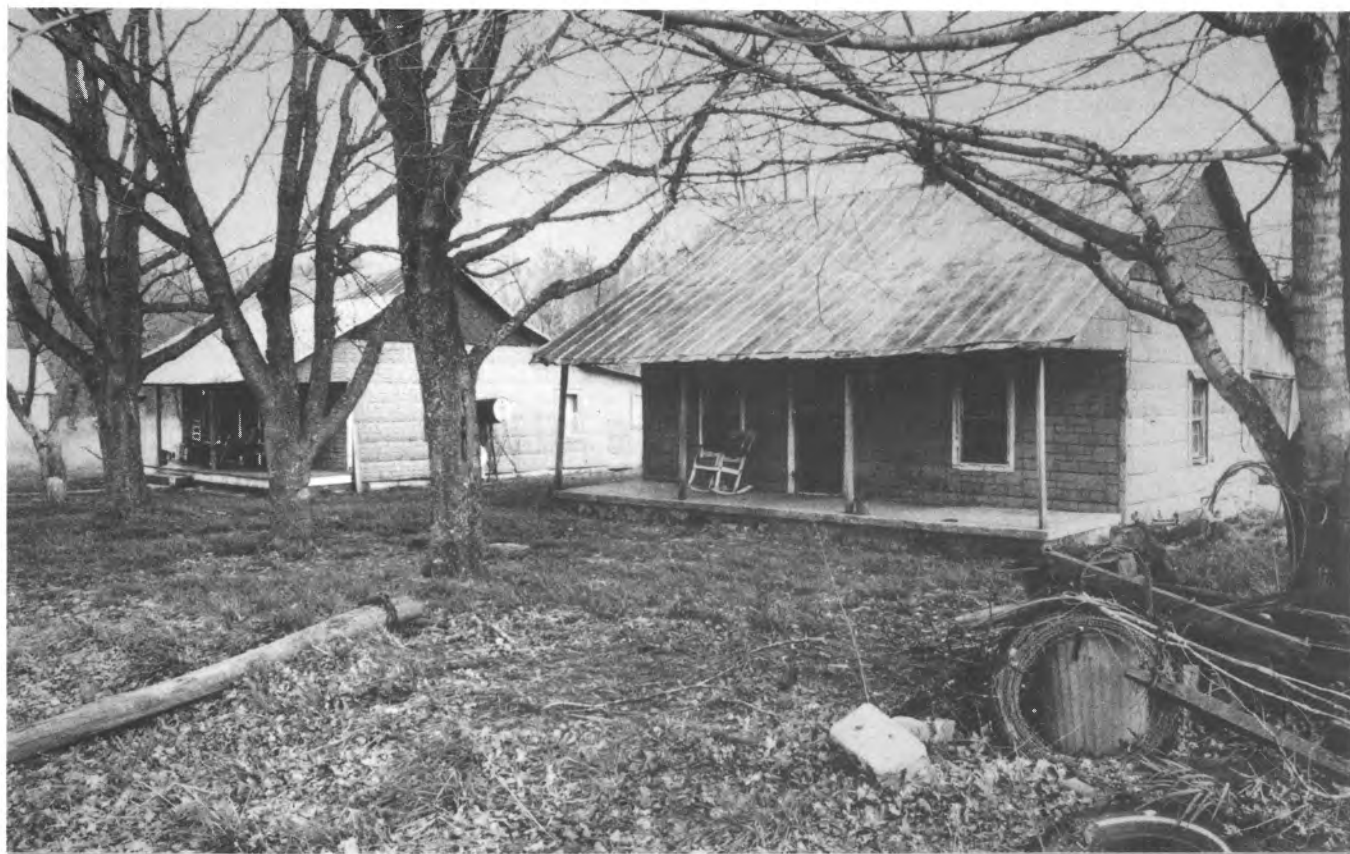
Figure 35. Cumberland Furnace Company House (Dickson County 329).
