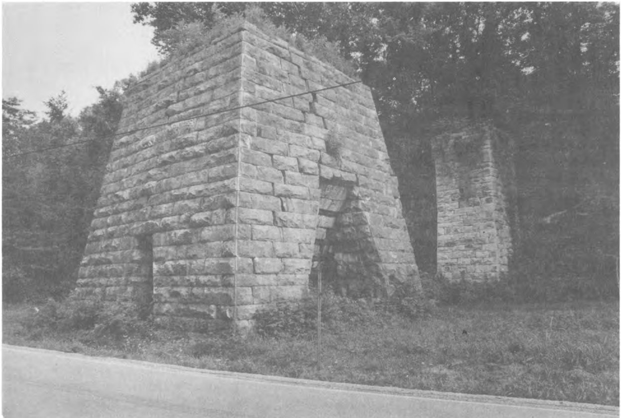
Figure 22. Remains of Bear Spring Furnace (40SW207).
