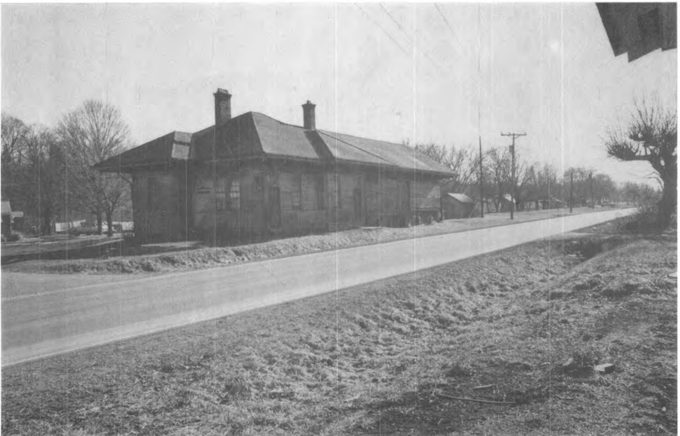
Figure 32. Cumberland Furnace Train Depot (Dickson County 325).
