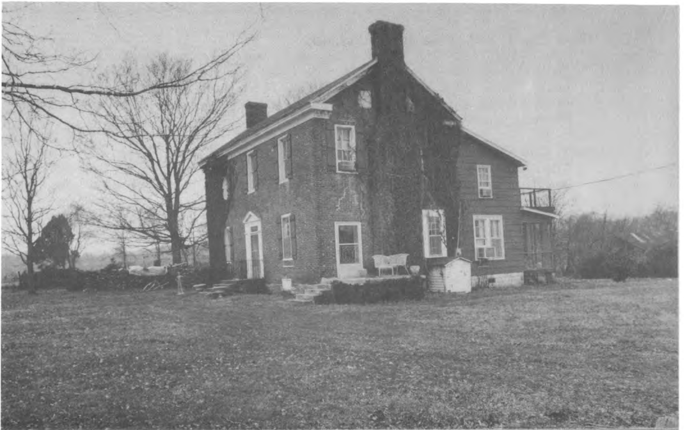
Figure 27. Napier House (Dickson County 319).
