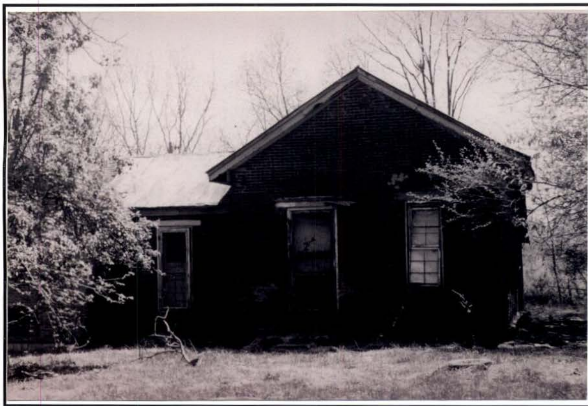
Figure 11. View of renovated antebellum “smokehouse”, looking south.
