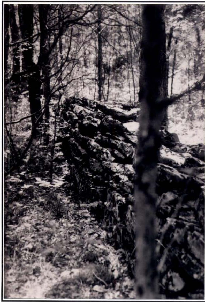
Figure 3a. Linear rock wall at 40RD222.
