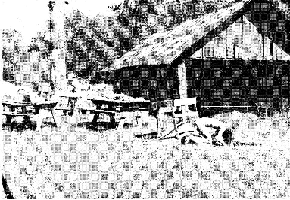
Figure 23. Cattle Weighing Barn.
