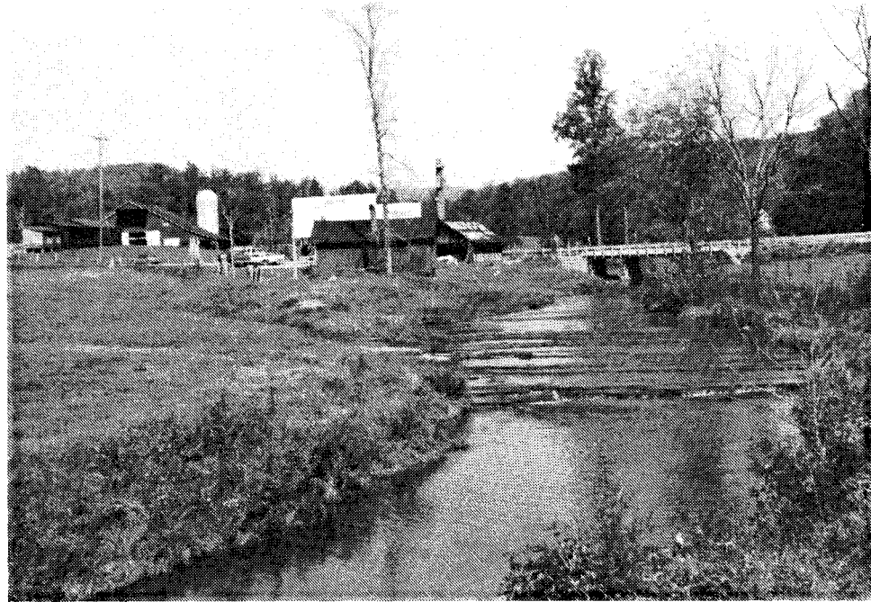
Figure 2. Caney Creek. View From Southern Tip of Site Looking North.
