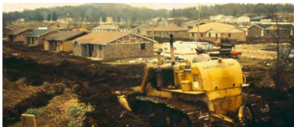
FIGURE 9. Spreading of mound fill across the residential development in 1984 (Courtesy, Mack Prichard).
