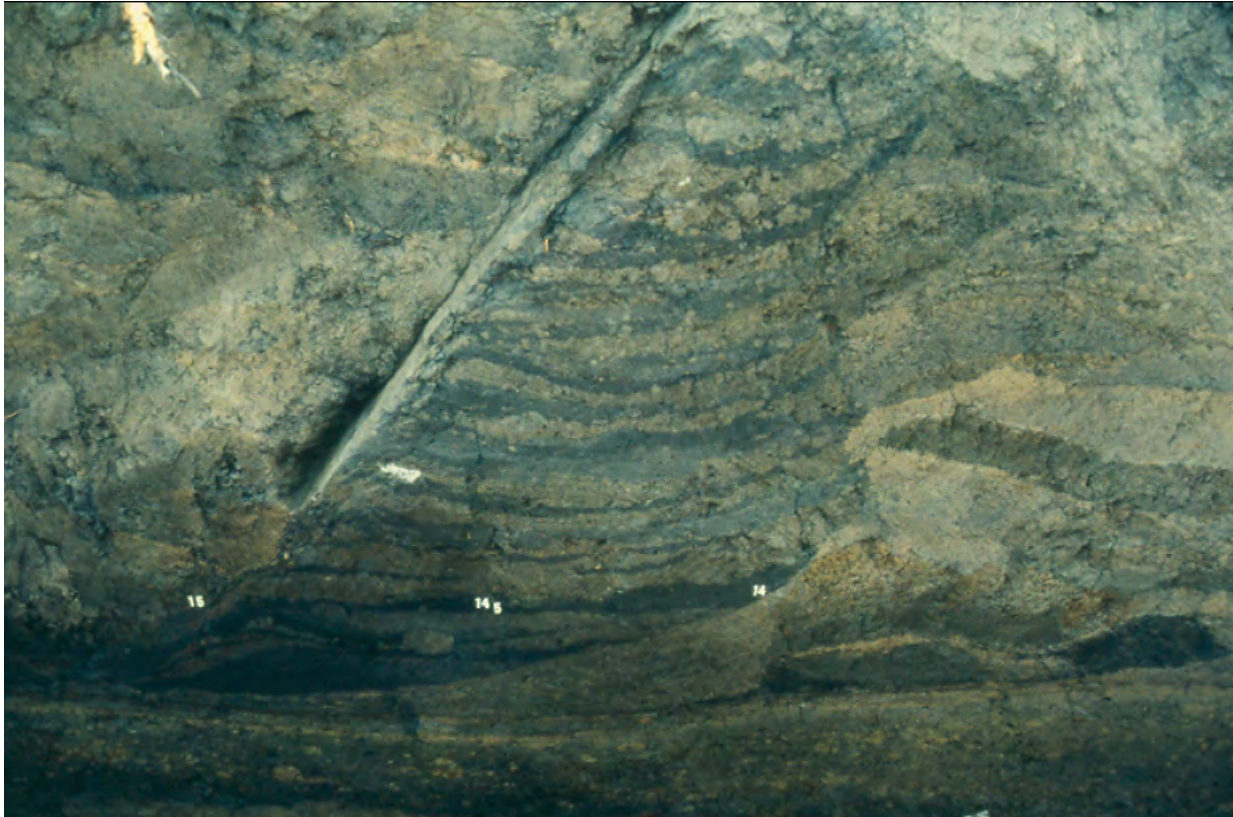
FIGURE 17. Profile of Stage II construction in Mound B showing distinct packed down basket loads of soil over Stage I. Note puddled clay layer over Stage II indicating additional stage(s) above it.
