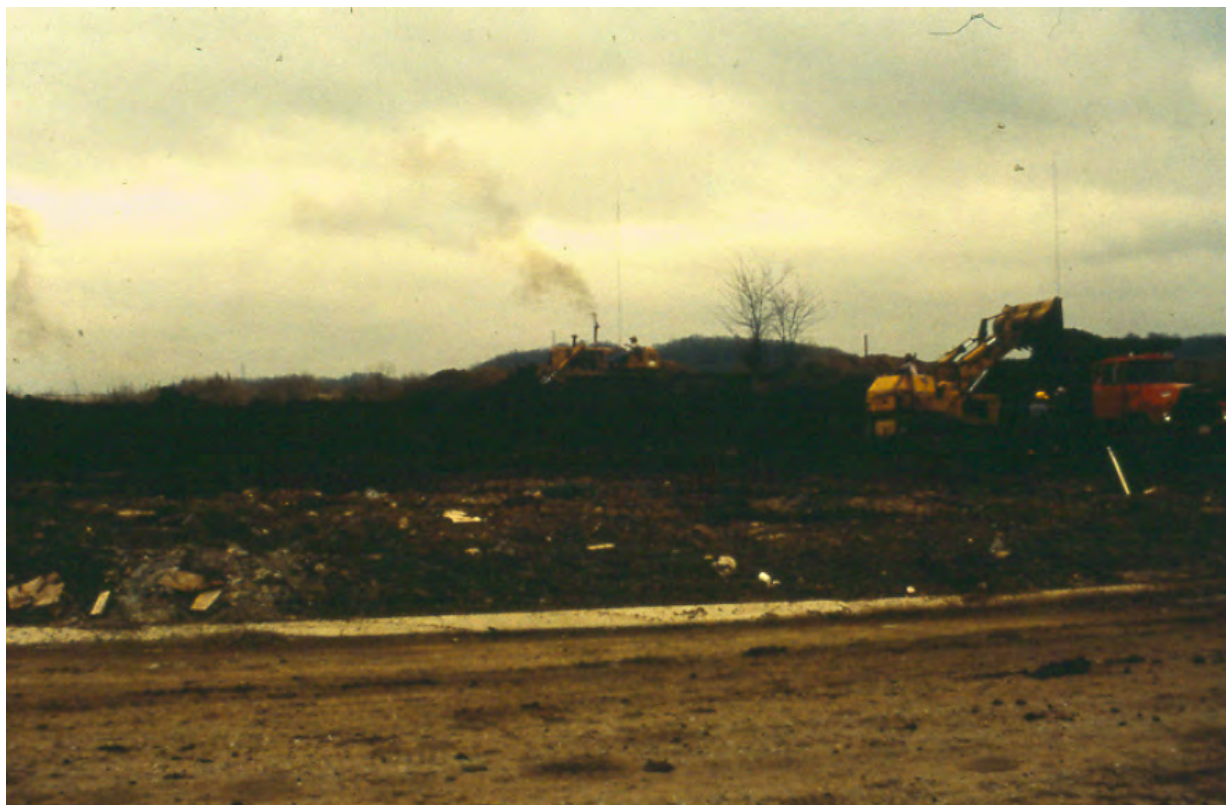
FIGURE 10. Leveling of the Brick Church Mound in 1984 (Courtesy, Mack Prichard).
