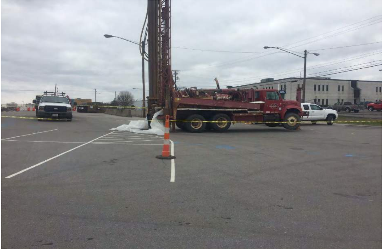
5. Drilling of planned MW-BNA01-01 location; boring abandoned, looking west
