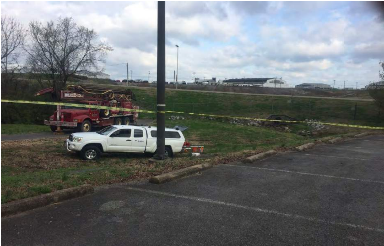
8. MW-BNA05-01 drilling, looking northwest
