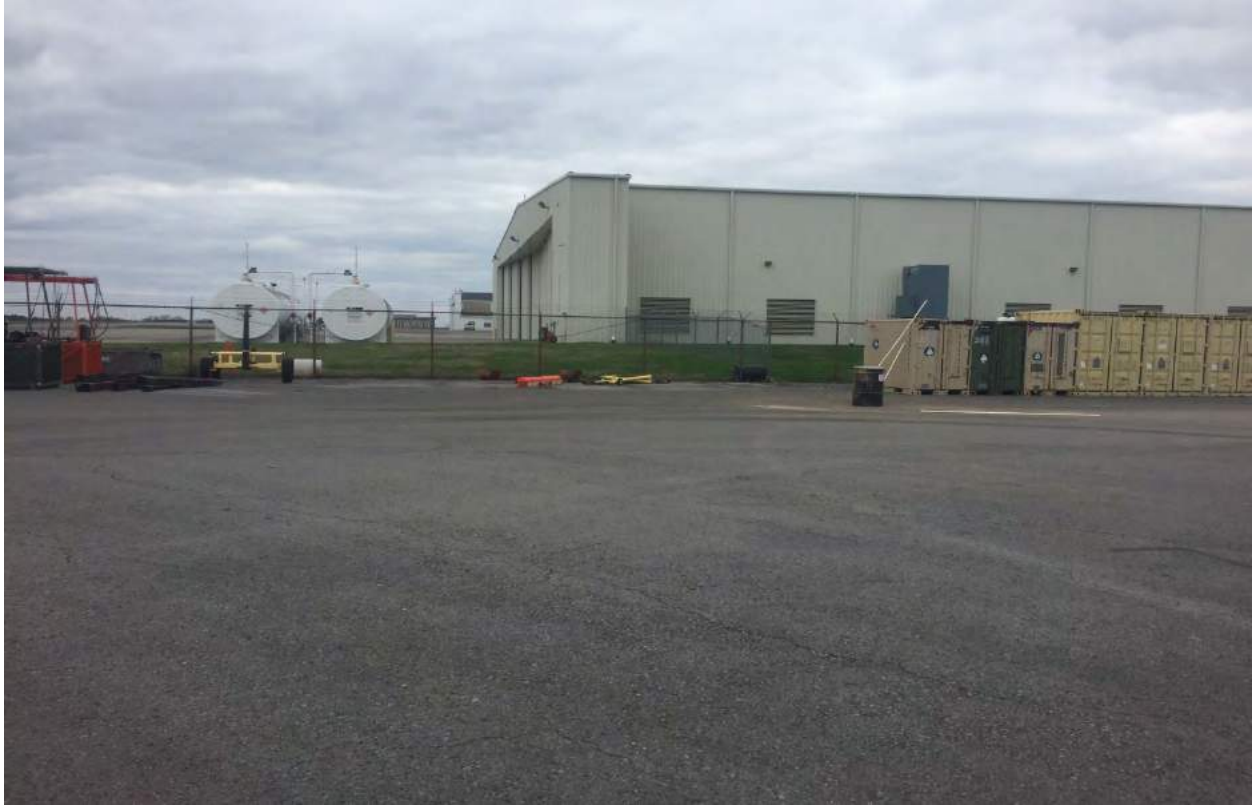
3. BNA03-SB2_PZ2 planned location, artesian, abandoned, looking west
