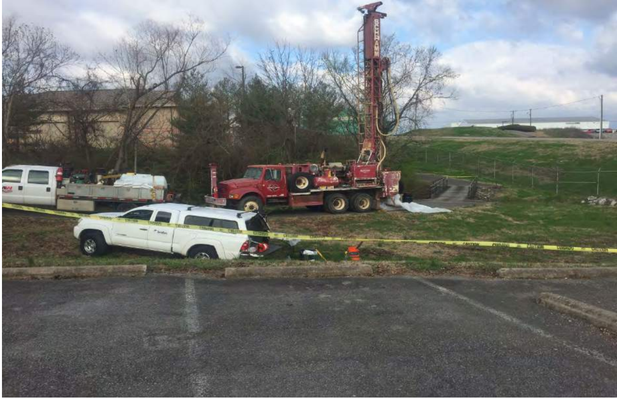
7. MW-BNA05-01 drilling, looking west (second view)
