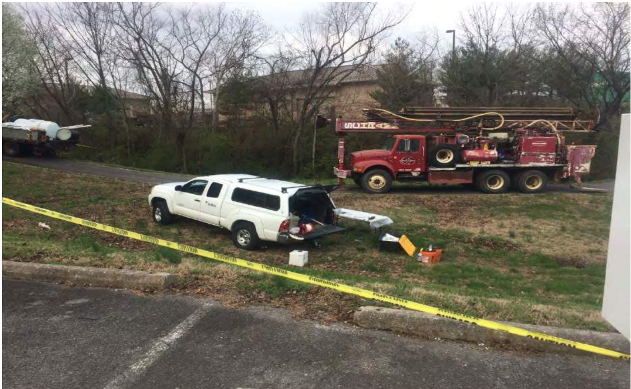
6. MW-BNA05-01 drilling, looking west (first view)
