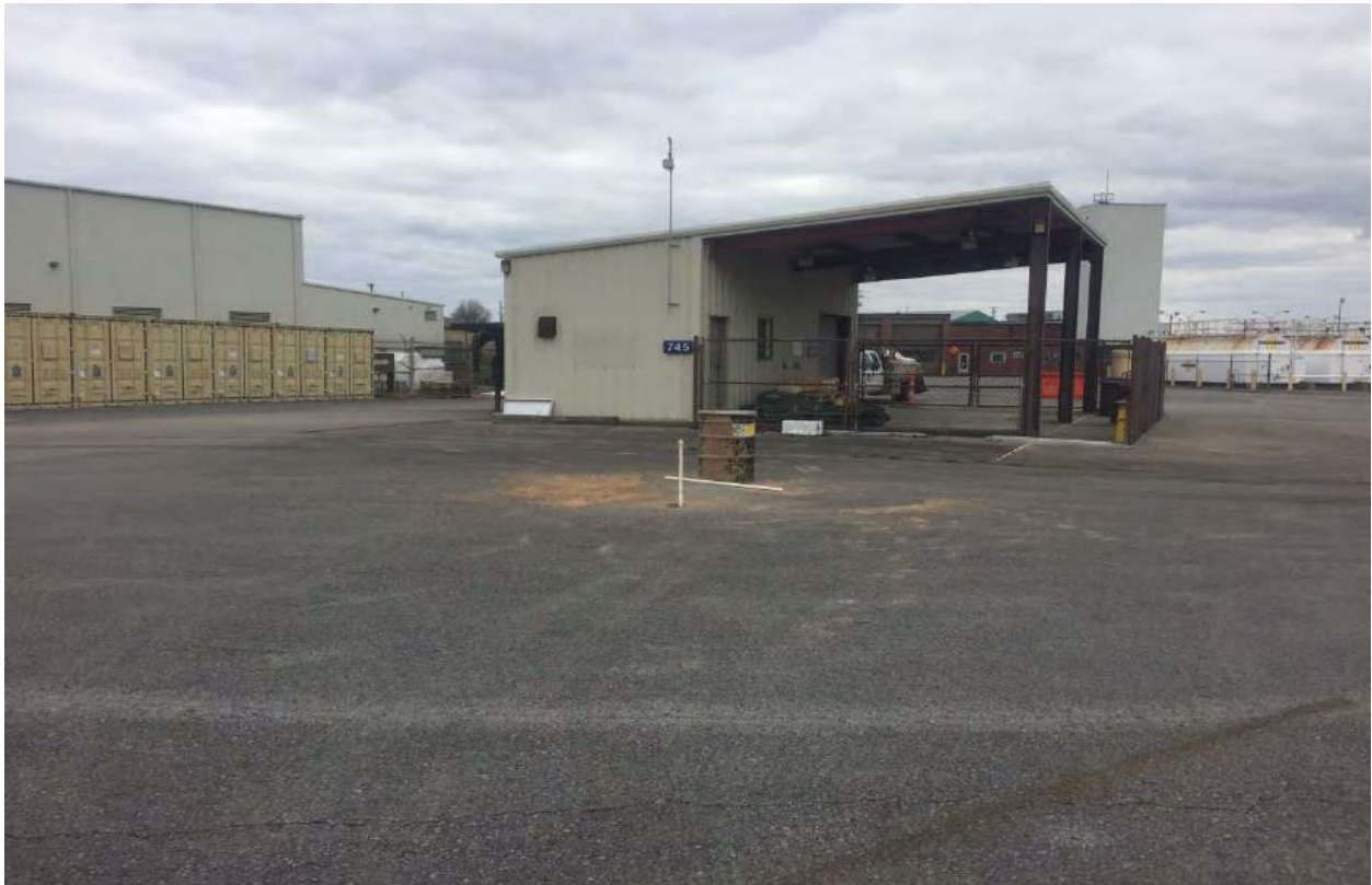
2. BNA03-SB2_PZ2 offset location, looking north-northwest
