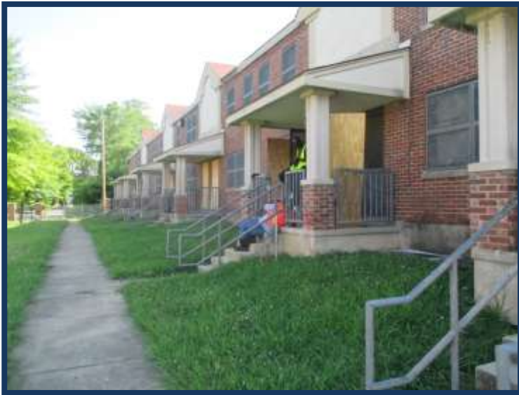
The boarded-up Foote Homes prior to demolition.
