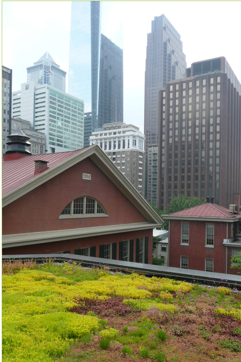
A green roof located on the Friends Center in downtown Philadelphia, Pennsylvania provides stormwater management capacity and adds aesthetic value to this dense urban environment.
