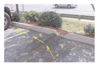
Site runoff bypasses bioretention swale because of small elevation changes during construction.
