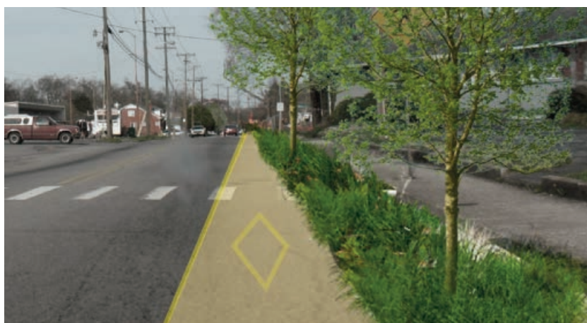
Figure 3.10: Conceptual representation of the same street retrofitted with linear bioretention, a bike lane, and street trees (Source: SMART Center).
