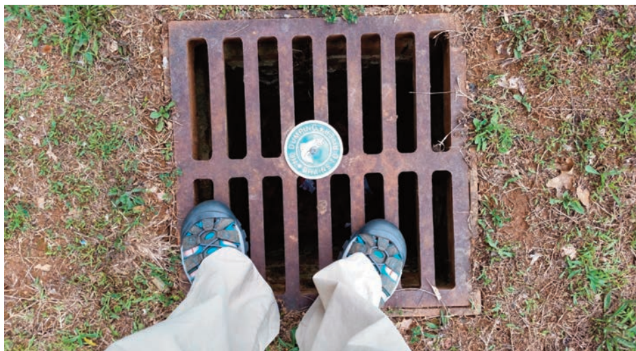
Figure 3.1: Stormwater management approach of storm drain stenciling, which identifies drains that discharge to local streams and states a no dumping regulation.
