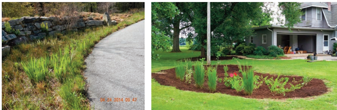
Figure 3.11: Photographs of lot scale runoff reduction measures. Left: a roadside vegetated verge (without curb or gutter) that accepts roadway runoff, uses engineered soils to infiltrate runoff, and conveys excess runoff to a small treatment wetland. Right: a residential rain garden captures and infiltrates runoff from the house rooftop and driveway.
