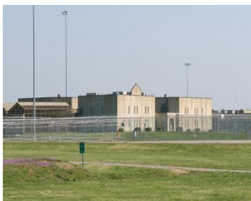
Northwest Correctional Complex
