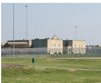
Northwest Correctional Complex
