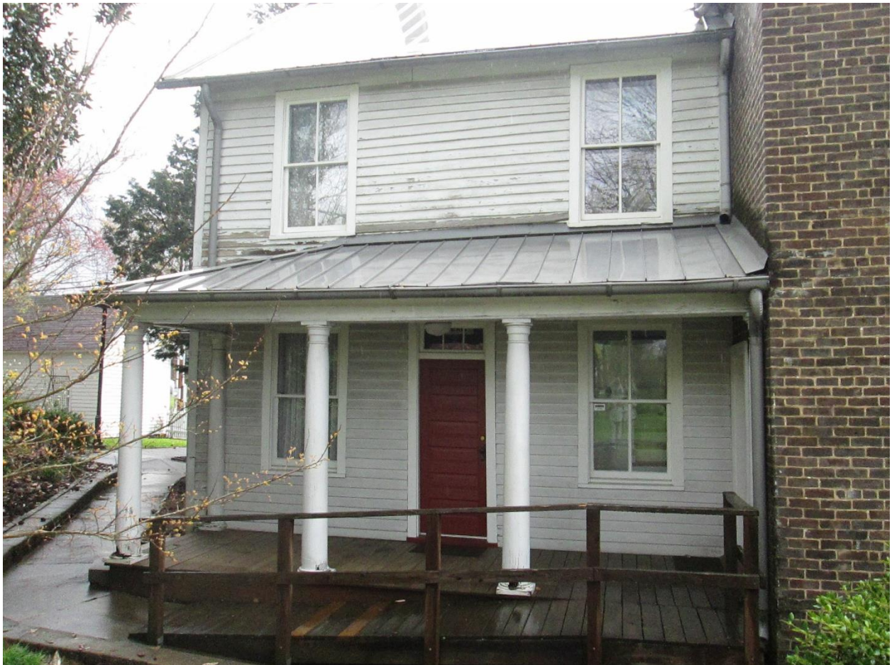
Photograph 1. Partial view of the west elevation of the Nance Building, facing east, showing the entire porch including the three freestanding columns and two pilasters.
