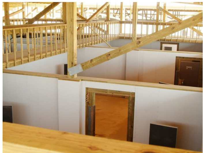
Shoot House at Olive Security Training Facility, Crawfordville, AR
