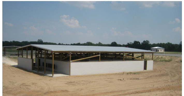
Shoot House at Olive Security Training Facility Crawfordville, AR
