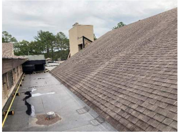
81) Roof – View of mechanical doghouse (left side) and typical shingle roof dormer providing clerestory lighting to main lobby.
