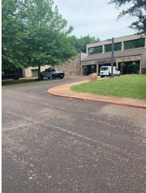
32) Path from Guest Rooms to Accessible Stalls
