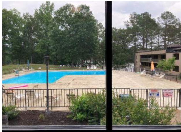
19) Lodge Exterior – Overview of the pool area from inside the dining addition.
