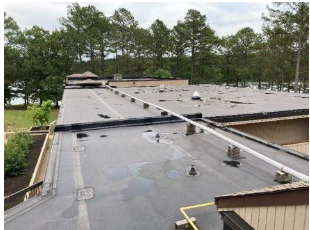
83) Roof – View of guest area.
