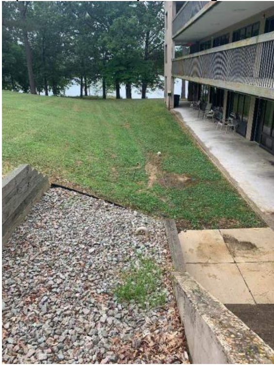
83) Pool Area – Inadequate Drainage
