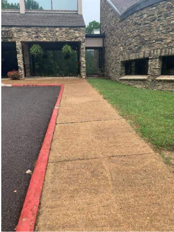
35) Path from Guest Rooms to Accessible Stalls
