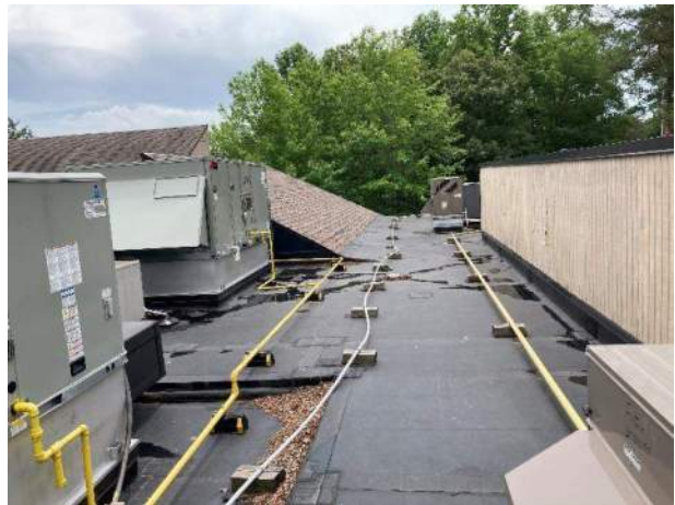
79) Roof – View of the area between conference and the kitchen.
