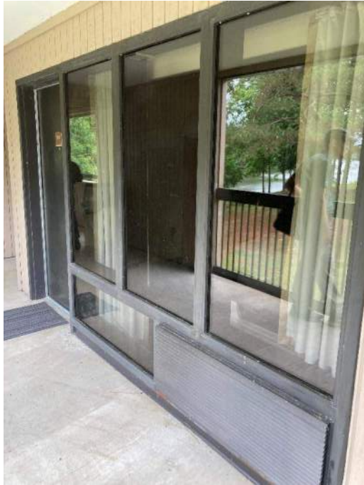
64) Typical Double Room – The 1990s stack of rooms have the original storefront and PTACs.
