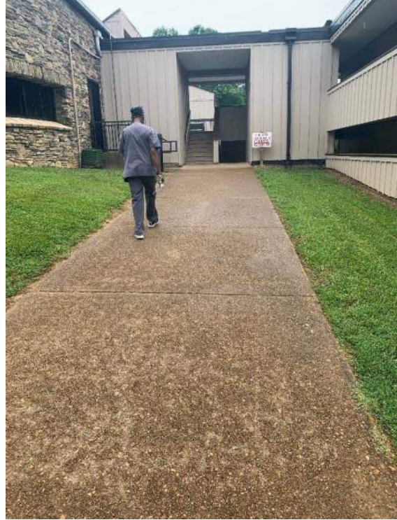
46) Sidewalk from Front Parking to Staircase
