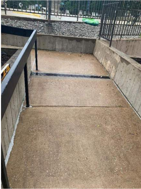
79) Pool Area – Inadequate Drainage
