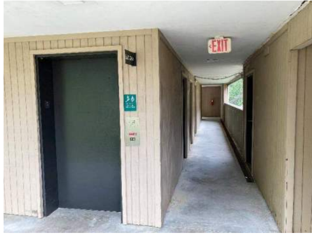
68) Guest Area – View of a typical exterior corridor, including the elevator which was added with the 1990s addition.
