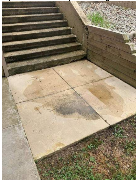
80) Pool Area – Inadequate Drainage
