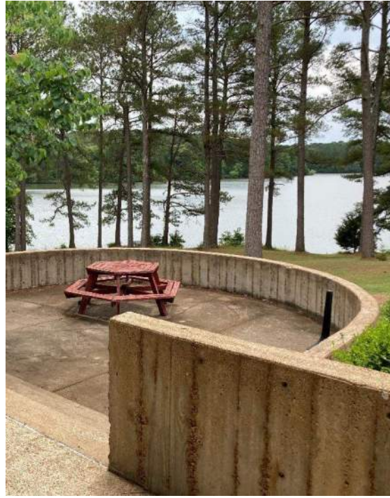
17) Lodge Exterior – Sitting areas on the South side of guest room. The State mentioned a desire to provide firepits in these areas.
