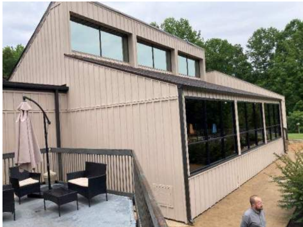
18) Lodge Exterior – View of the dining addition. Siding has been replaced in this area with board and batten siding.
