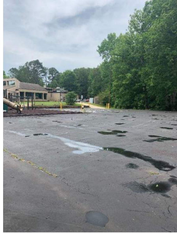
89) Rear Parking Lot Drainage
