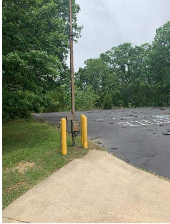
90) Rear Parking Lot Drainage
