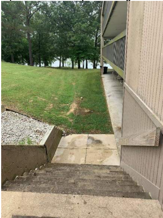
79) Pool Area – Inadequate Drainage
