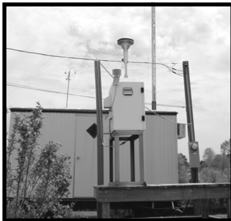
Hazardous Air Pollutants Monitor, Loudon County, Tennessee. Source: David Borowski, Tennessee Department of Health.
