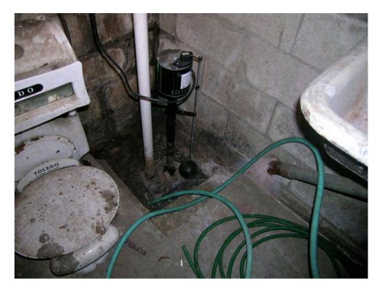
**Photo 5** - View of sump in the northwest corner of the basement of Home A. There is an identical sump pump in the southwest corner of the basement. (Photo credit: TDH, 04/18/11).
