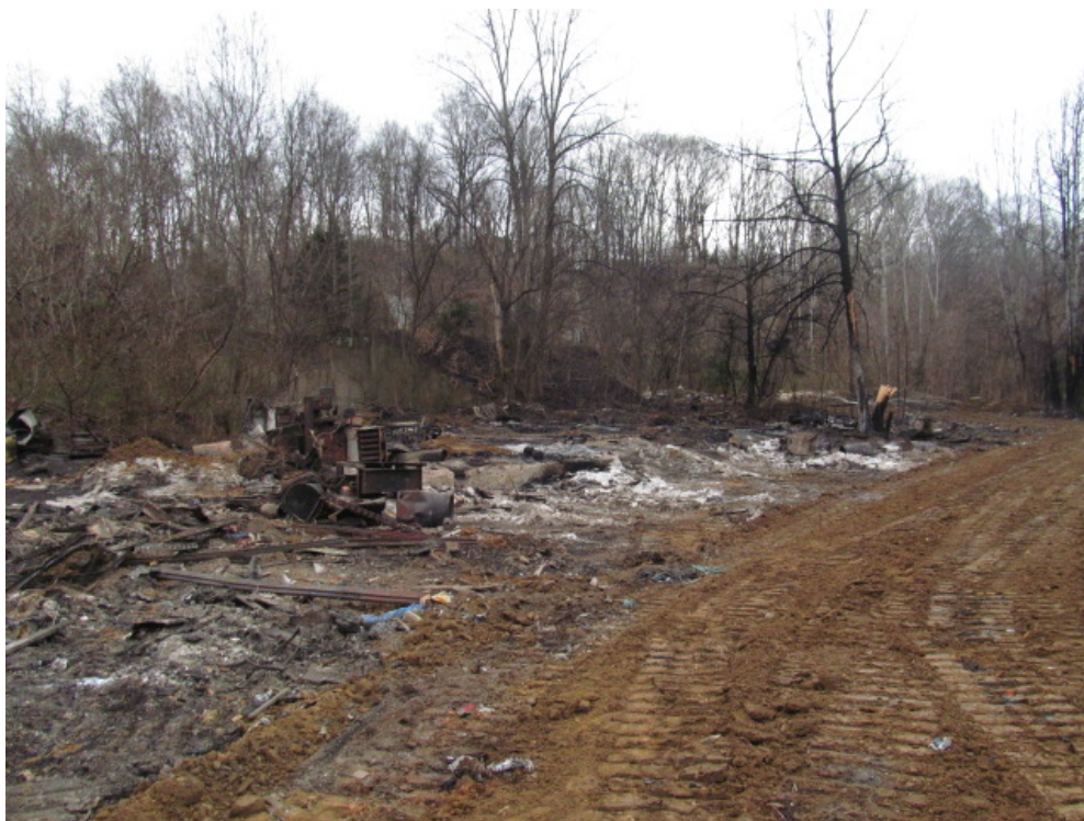
View of burned plastic and debris along North Fork of Mill Creek on property on December 21, 2013 after the fire was smothered. View is toward the south-southwest. Source: EPA.
