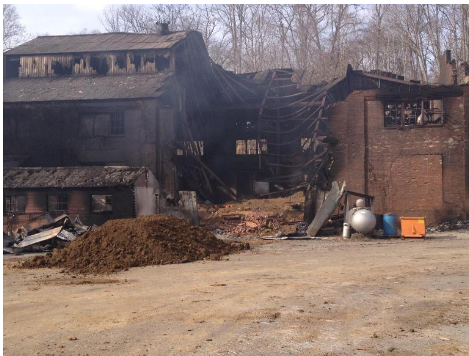
Onsite building burning on December 19, 2013. Note soil stockpiles to be placed on fire burning inside the building. Note the absence of structural integrity of the building. View is to the northeast. Source: EPA.
