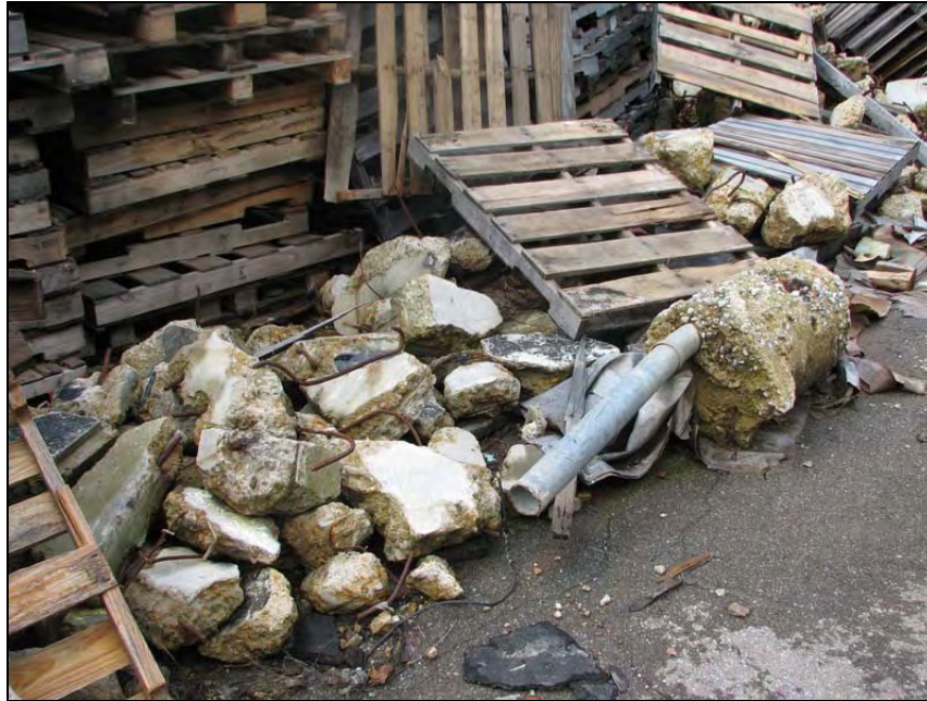
Figure 13. Mounds of concrete and wooden pallets on Tax Parcel 167C H 002 of the Oakland Avenue and 45 th Street (Alton Park Area 3) site, Chattanooga, Hamilton County, TN. (Photo credit: Sarah Stuart Chewning and Sabrina Novak, Chattanooga-Hamilton County Health Department – 5/7/09)
