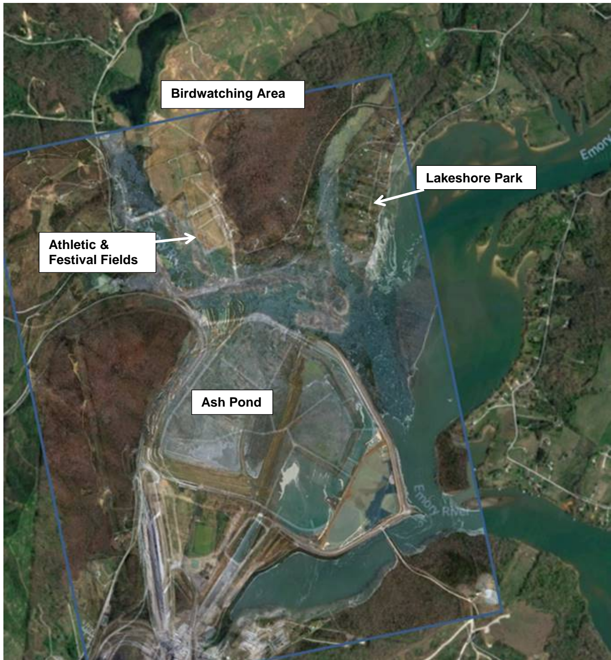
Figure 3. Overlay of the extent of TVA Coal Ash Release with the closed coal ash pond and Athletic & Festival Fields, Birdwatching Area, and Lakeshore Park areas noted.
