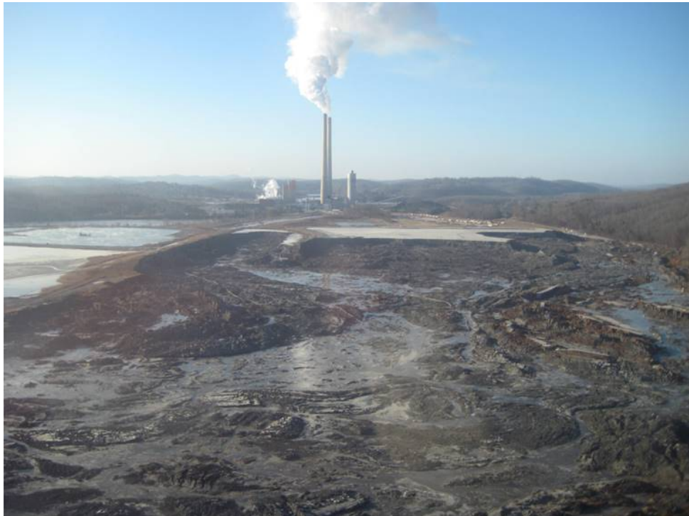
Figure 1. TVA's Kingston Coal Ash Release in December 2008. View is looking south at the breached containment dike area. Note the coal ash spilled into the Emory River toward where Roane County's Swan Pond Sports Complex is now located. Image source: TVA
