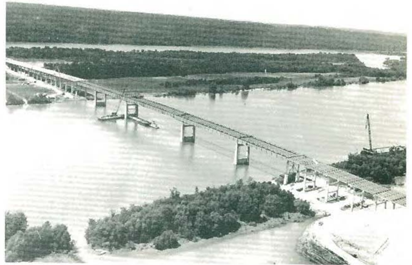
Work was started on the 4.2 mile long Tennessee River Bridge on November 29, 1962. This four-lane facility spanned the historic boundary between Middle and West Tennessee. To close the gap between these two geographic sections, thousands of man-hours in labor and tons of concrete and steel were required.
