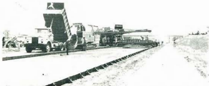
This concrete paving train and spreader were in the process of completing paving on Interstate 40 near Nashville. Scenes similar to the above were frequent as workmen rushed to complete this important segment of Interstate highway between Nashville and Memphis.
