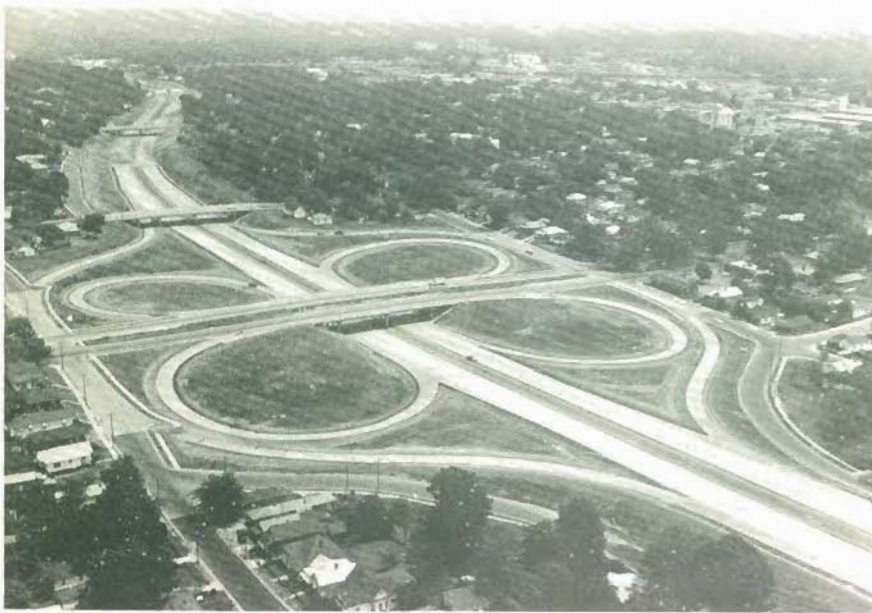
I-255 and East Parkway Interchange in Memphis.
