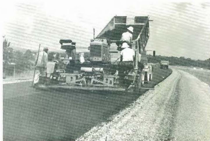
Workmen on this asphalt paver above were taking advantage of the fine summer weather to complete work on a section of Interstate highway which connects Memphis and Nashville, I-40 greatly reduces driving time between the two cities. Shoulders also were in process of being finished for emergency stopping.
