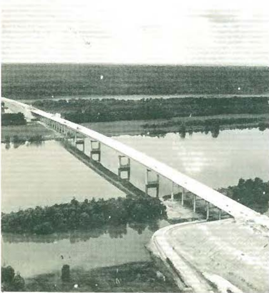
The Tennessee River Bridge was almost three years in construction and was finally completed on July 21, 1965.
