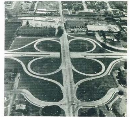
I-75 and Baxter Avenue Interchange in Knoxville.
