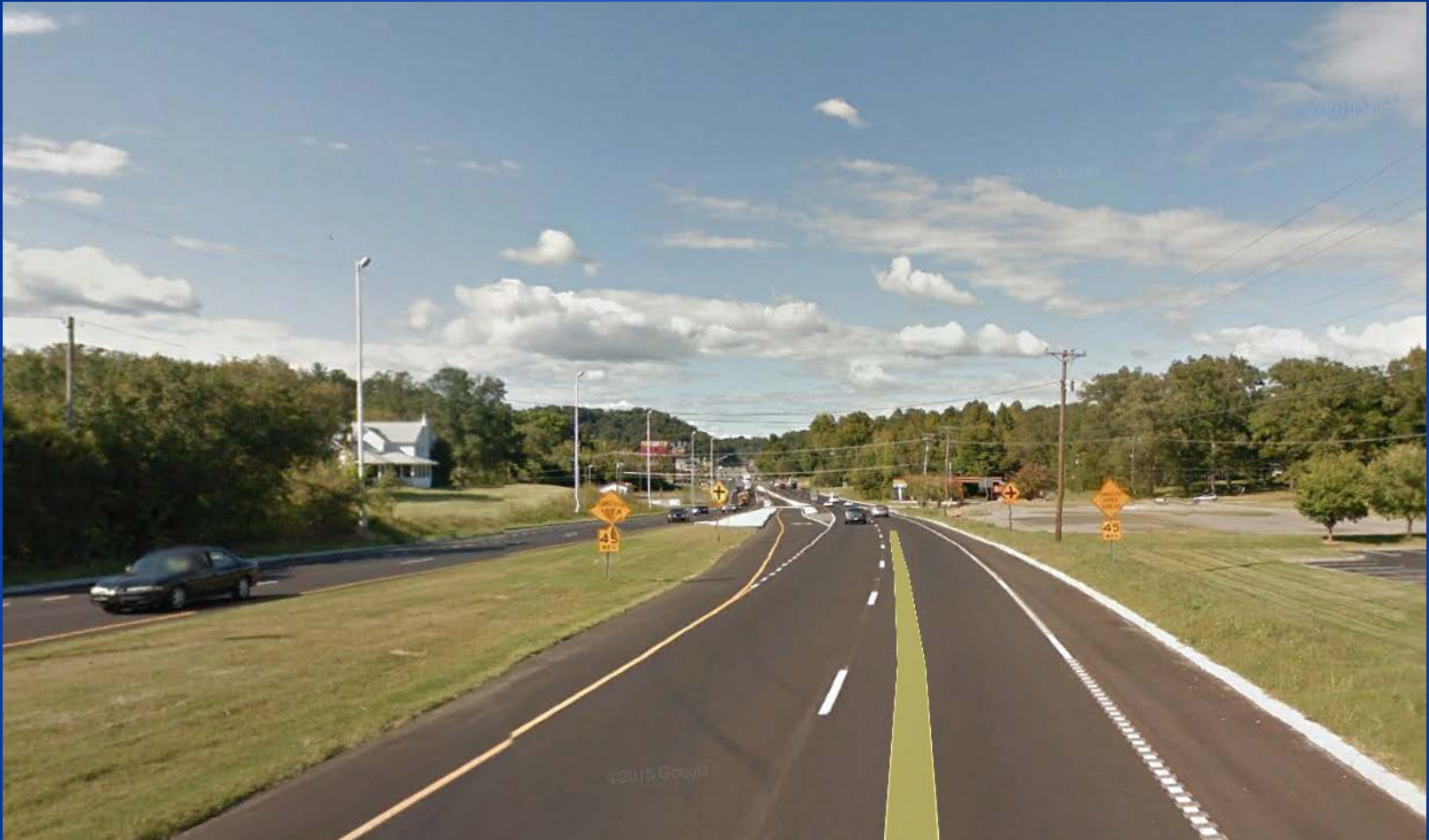
Existing SR 115 (US 129) Alcoa Hwy
