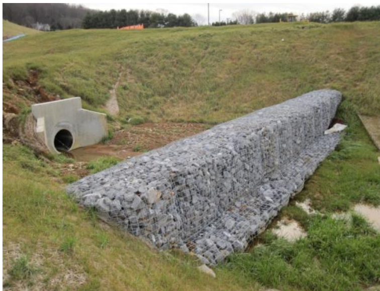
Figure 7.31-2C Forebay with Porous Berm (Gabion Rock)
