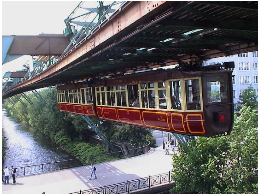
Figure 2: Schwebebahn in Wuppertal, Germany
