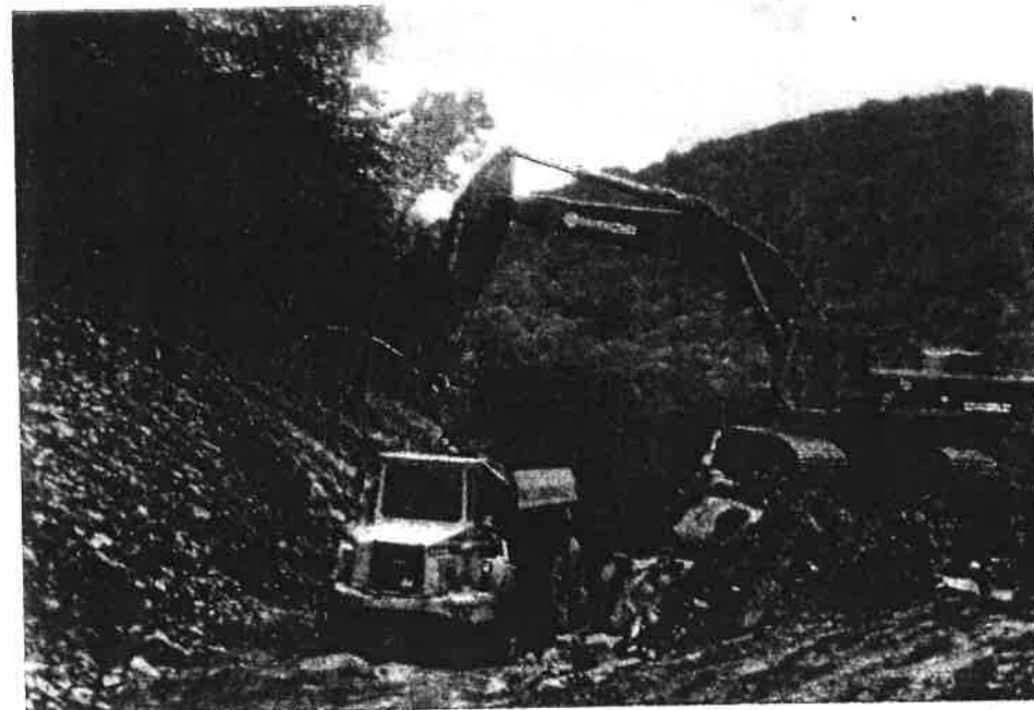
Recent construction on the North Carolina portion of the Skyway.
