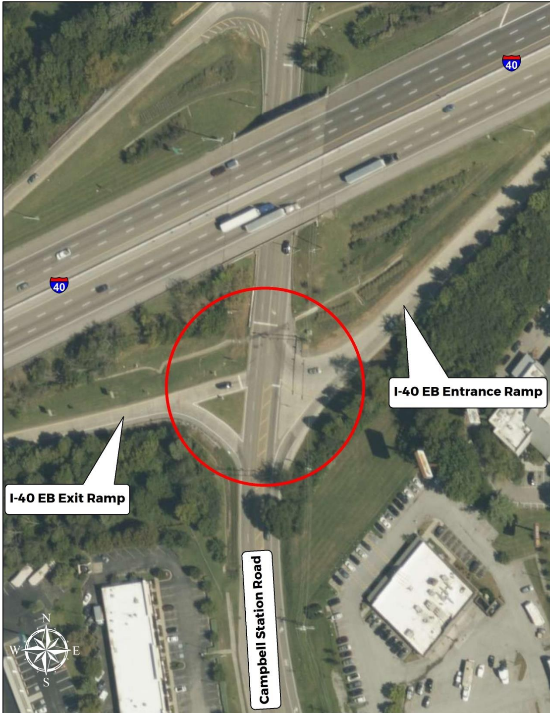
Figure 8. I-40 Eastbound Ramps at Campbell Station Road
