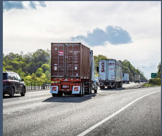
Climbing lanes are recommended in several locations along the corridor where trucks are slowed by steep terrain.
