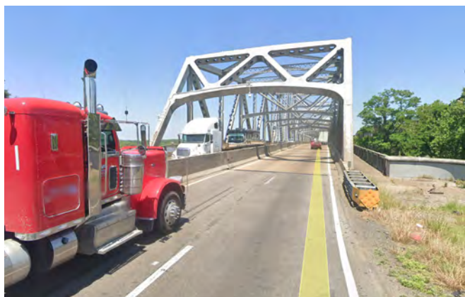
Figure 4-3. I-55 WB Approaching Mississippi River Bridge
