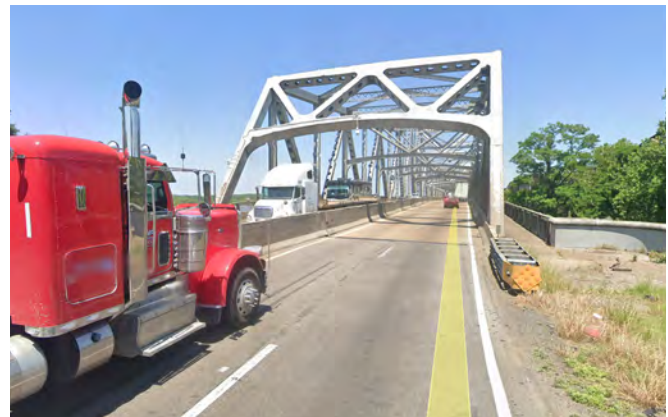
I-55 WB approaching Mississippi River Bridge
