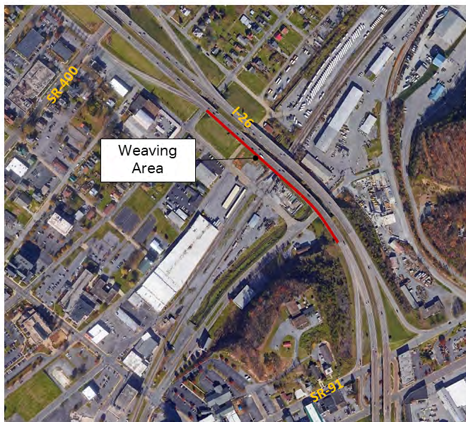
Eastbound weave area between SR-400 and SR-91
