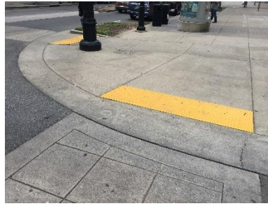
Example Parallel Curb Ramp
