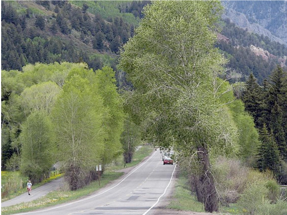
EXHIBIT 2-10: RURAL ROAD WITH SEPARATED SHARED-USE PATH
