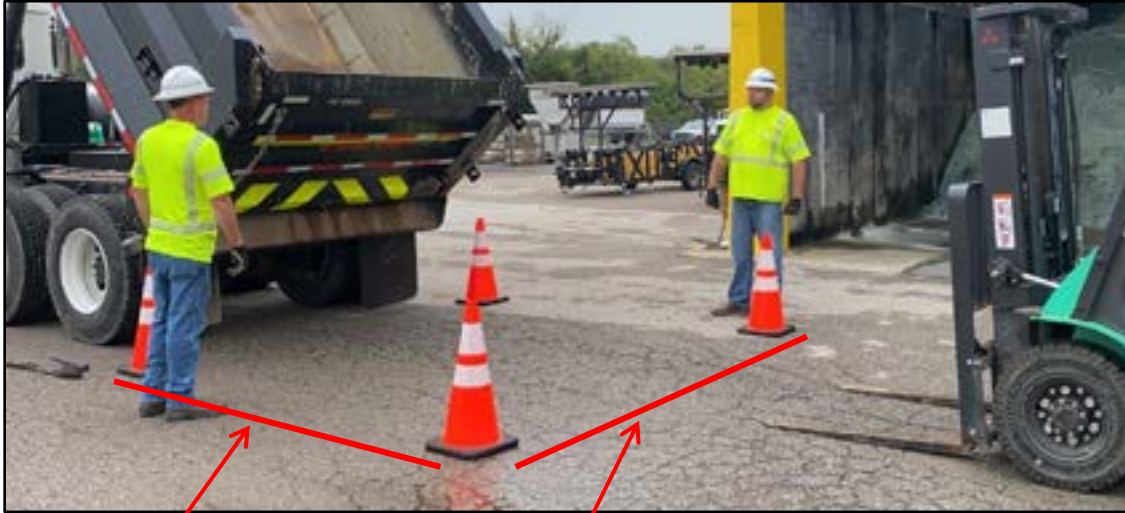
Photo A, A1 – Cone placement. Delineates work area.
