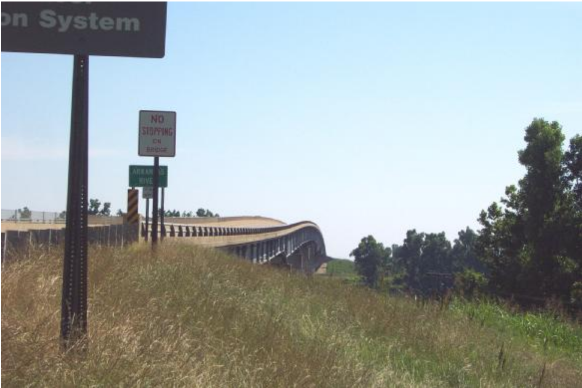
Hwy 79 at Arkansas River Crossing
