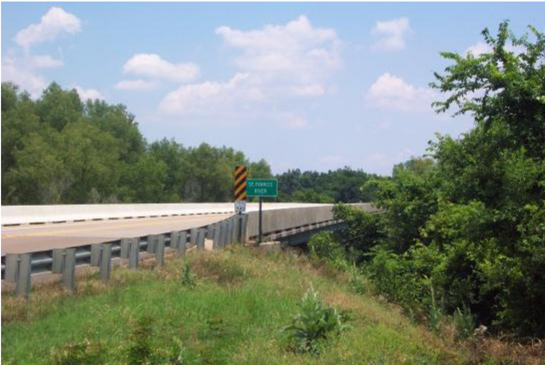
Hwy 79 at the St. Francis River
