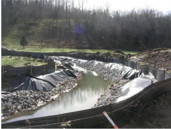
Temporary Diversion Channel Location: SR-15, Hardin County, TN (2004)
