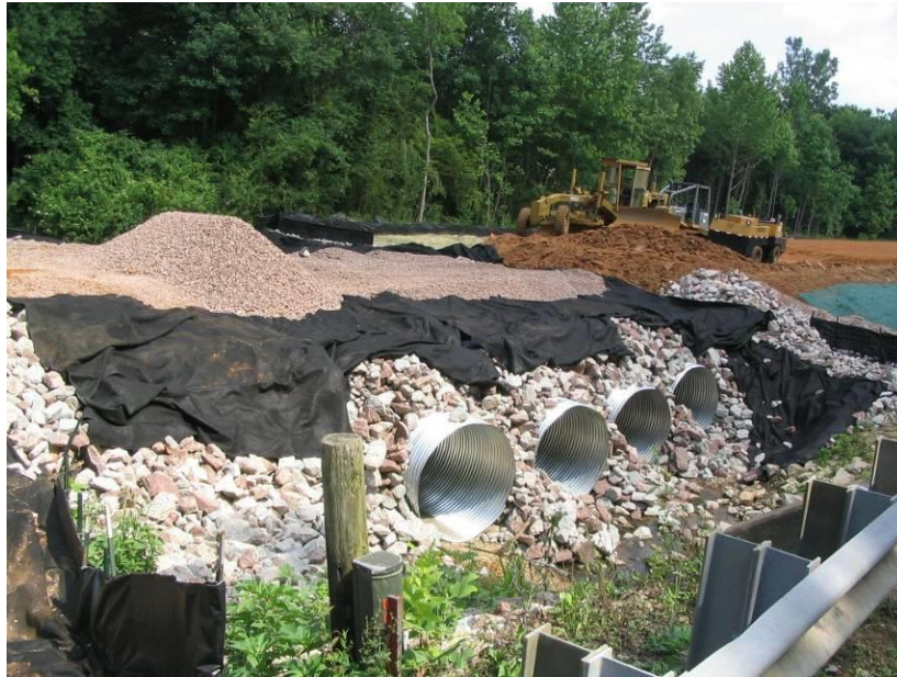
Multiple Pipes at Temporary Culvert Crossing Location: SR-224, McNairy County, TN (2005)
