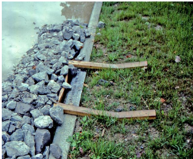
Curb Inlet Protection Type 3
