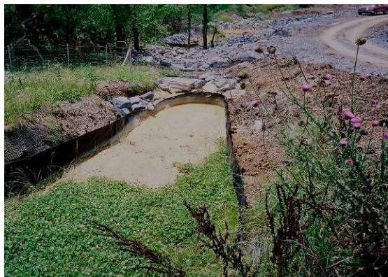
Enhanced Silt Fence Reference: SR-840, Williamson Co., TN (2004)
