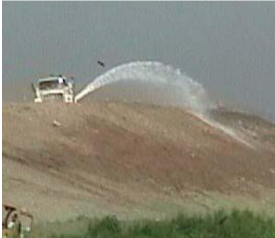
Applied Soil Stabilization Photo courtesy of Caltrans Guidance for Temporary Soil Stabilization (2003)
