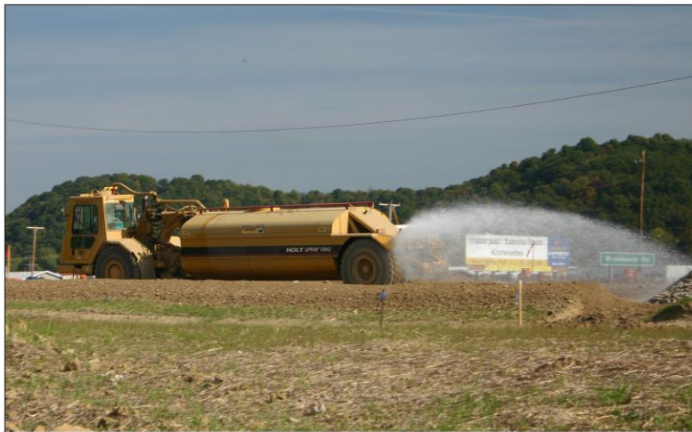
Figure 10-8 Watering the Construction Site for Dust Control Reference: Ohio DNR (2005)
