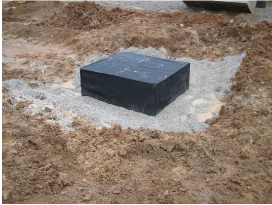
Catch Basin Filter Assembly on Inlet Location: SR-840, Williamson County, TN (2004)
