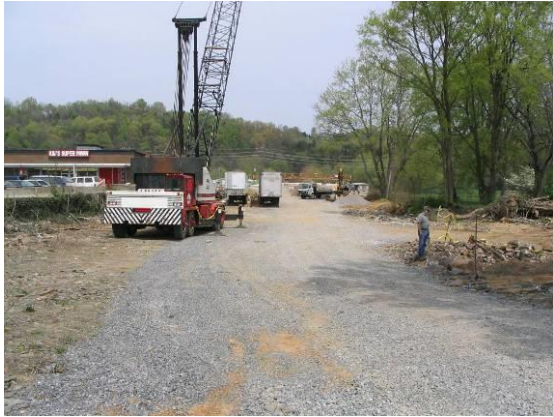
Temporary Construction Exit Location: SR-448, Sevier County, TN (2005)
