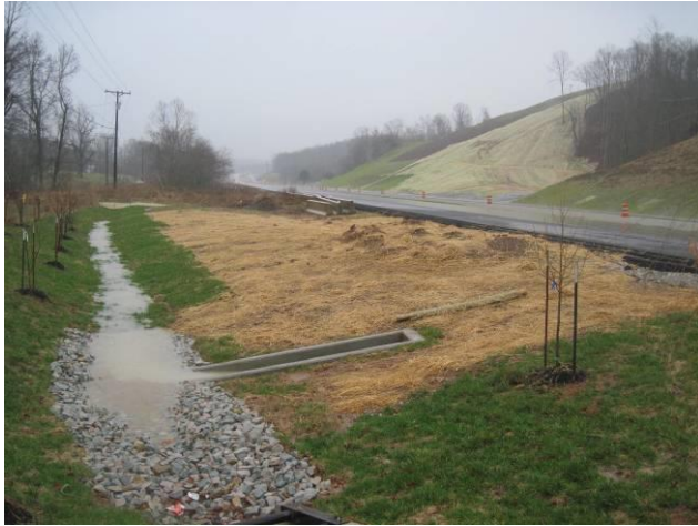
Applied Seeding with Mulch Location: SR-15/US-64, Wayne County, TN (2011)
