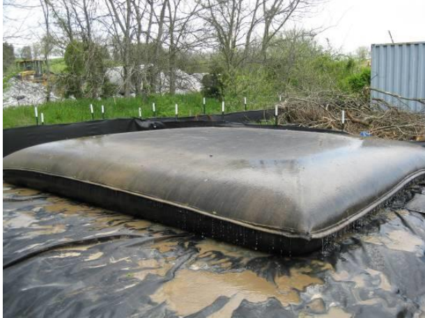
Sediment Filter Bag With Silt Fence & Stream Buffer
