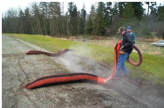
Filter Socks in Ditch Application Reference: Filtrexx International, LLC
