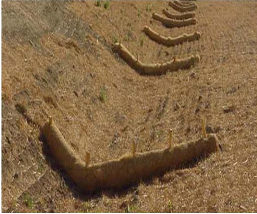
Sediment Tubes in V-Ditch Application Reference: Colorado DOT, (2002)
