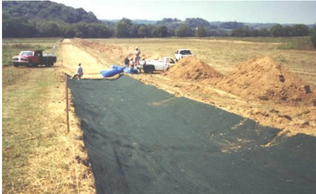
Turf Reinforcement Mat Location: SR 840, Williamson County, TN (2004)
