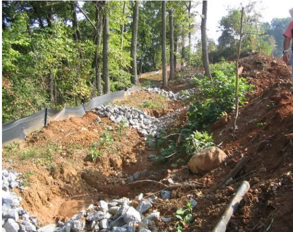
Installation of Rock Check Dams Location: SR-37, Carter County, TN (2004)
