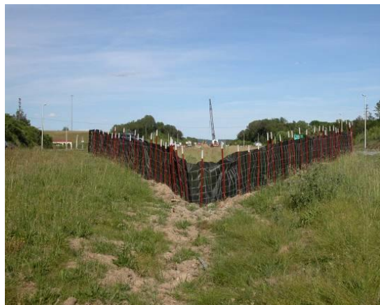
Enhanced Silt Fence Check Location: I-40, Smith County, TN (2005)
