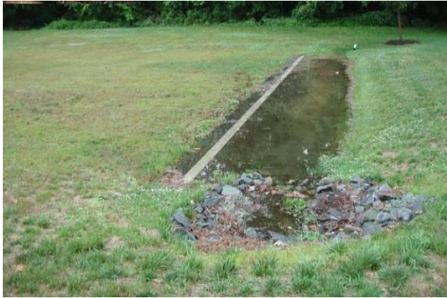
Constructed Level Spreader (Type 3) Source: BEA Group at NC State University
