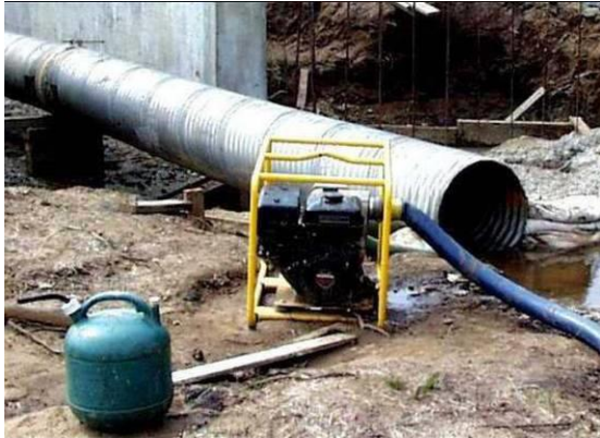
Suspended Pipe Diversion Source: NCDOT (2003)
