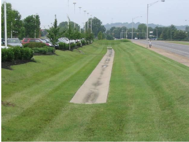
Permanent Detention Basin w/ Low-Flow Concrete Trickle Ditch for Drainage Location: US-41, Nashville, TN (2006)
