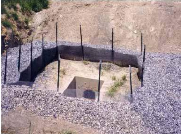
Catch Basin Protection (Type B)
