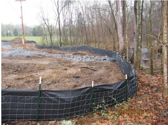
Silt Fence with Wire Backing Location: SR-250, Cheatham County, TN (2007)
