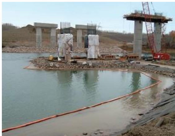
Floating Turbidity Curtain Used at Bridge Crossing Reference: North Carolina DOT
