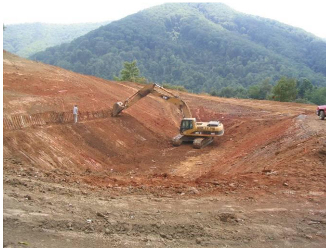
Figure 10FC-2 Permanent Detention Basin under Construction Location: SR-37, Carter County, TN (2005)
