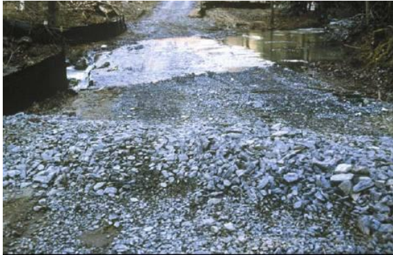
Temporary Construction Ford Reference: NCDOT (2003)
