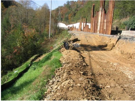
Temporary Berm at Top of Fill Slope Location: SR-73, Sevier County, TN (2004)
