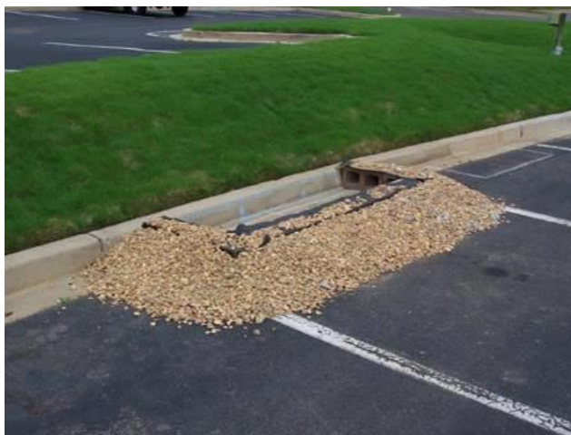
Type 1 Curb Inlet Protection Type 1 (Block and Gravel) Reference: International Erosion Control Association Photo Gallery, (2001)
