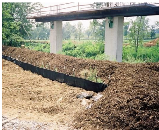
Mulch Berm with Silt Fence Location: SR-840, Williamson County, TN
