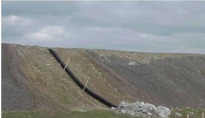
Temporary Slope Drain Reference: Handbook for Sediment and Erosion Control, Ohio DOT (2000)
