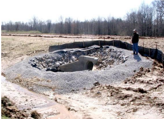
Installation of Culvert Protection Type 1 Location: SR-385, Memphis, TN (2005)
