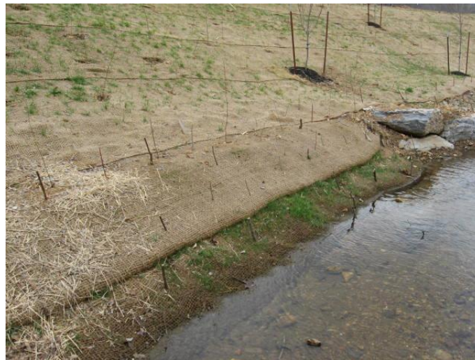
Figure 11SB-1 Live Stakes Placed at Outside of Channel Bend Location: SR-15, Furnace Branch, Wayne Co., TN (2011)
