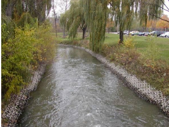
Vegetated Articulated Block Protection Location: Pennsylvania
