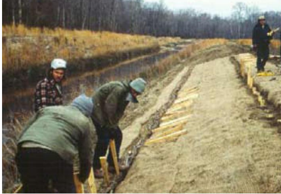
Live Fascines Installation
