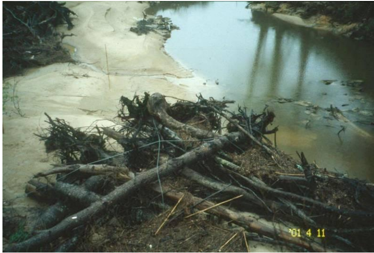
Figure 11HC-13 Engineered Rack Structure Installation Location: Topashaw Creek, Mississippi (2001)
