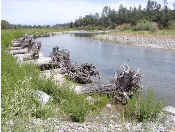
Root Wad Revetment Location: Clear Creek, Redding, CA
