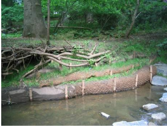
Coconut Fiber (Coir) Rolls Reference: Montgomery Co., MD DEP (2005)
