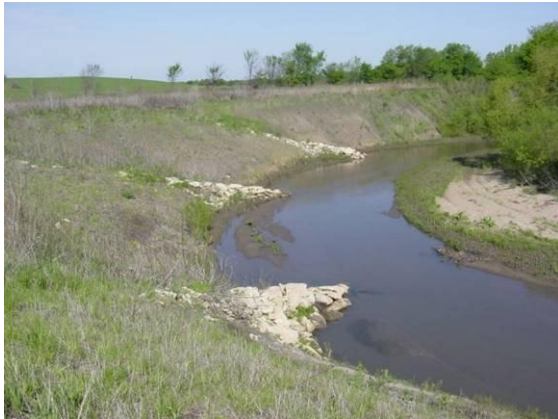
Spur Dike Installation Reference: USDOT, FHWA
