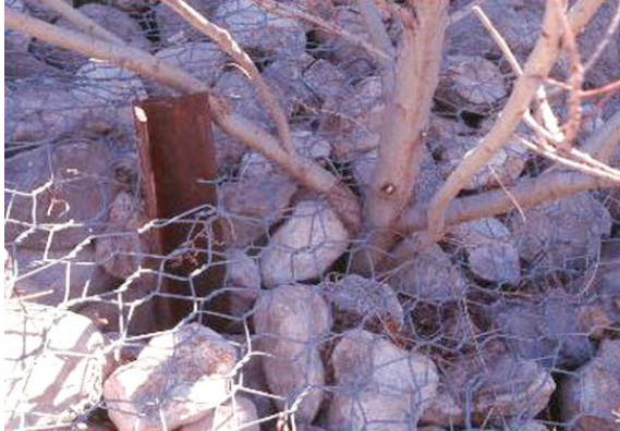
Gabion with Willow Tree Reference: GA DNR-CRD, (2006)
