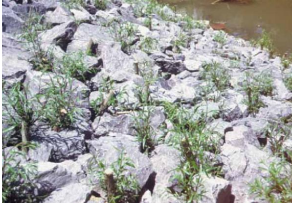
Vegetated Riprap along Stream Bank Reference: NRCS, Engineering Field Handbook 6
