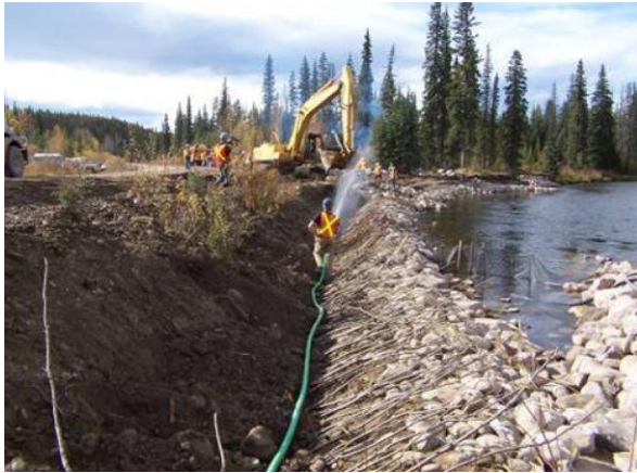
Live Siltation Construction Location: Pembina River, Alberta, Canada
