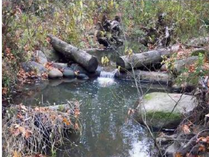
Figure 11HC-4 Typical “K” Weir Installation Reference: Washington Dept. of Fish and Wildlife, 2004 Stream Habitat Restoration Guidelines, Final Draft
