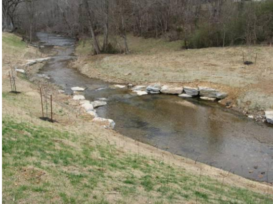
Cross Vane in Reconstructed Stream Location: SR-15, Wayne County, TN (2011)
