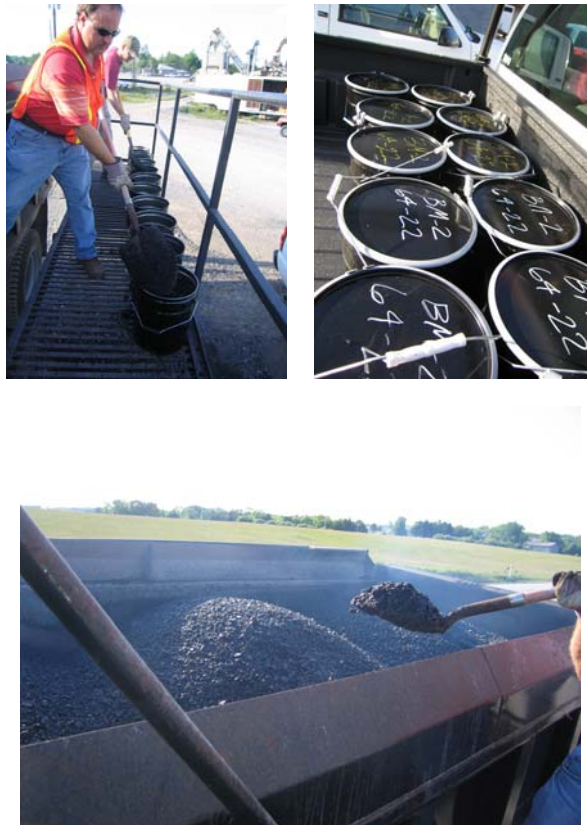
Figure 3.1 Field Collection of HMA Samples
