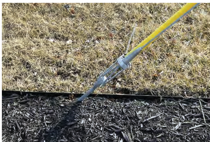
Figure 26. Example of a breakaway guy wire (Source: Delaware DOT).
