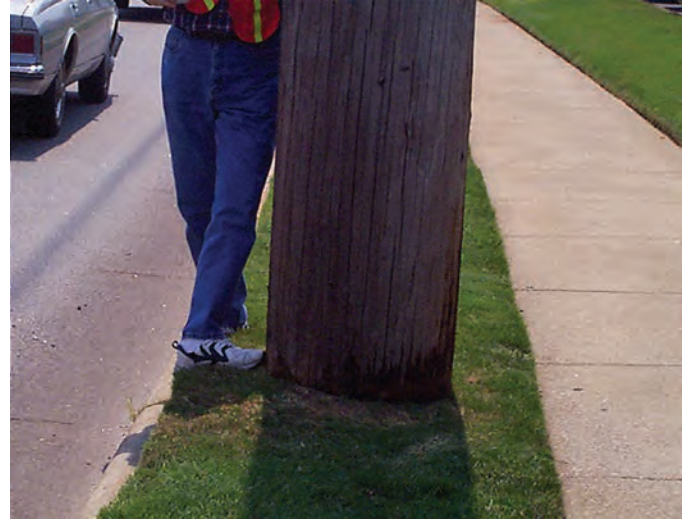
Figure 15. Examples of high-risk poles too close to the roadway (Photos: Charles Zegeer).
