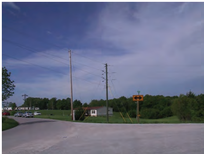
Figure 17. Example where pole relocation can greatly reduce the risk of utility pole crashes, at the top of a T-Intersection (Photo: Charles Zegeer).
