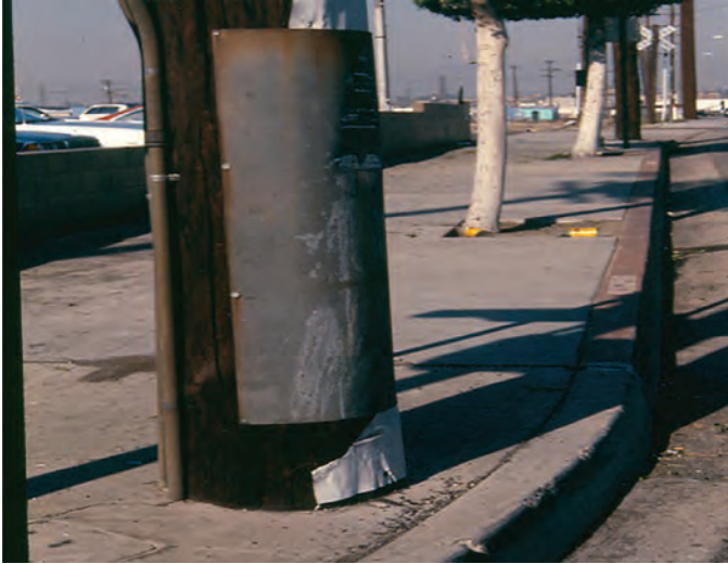
Figure 15. Examples of high-risk poles too close to the roadway (Photos: Charles Zegeer).
