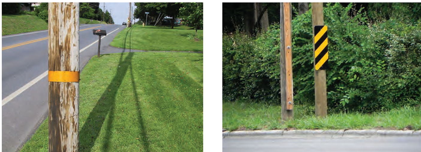
Figure 27. Examples of reflective tape on utility pole (left) and reflective panel (right) (Photos: Kevin Zegeer).
