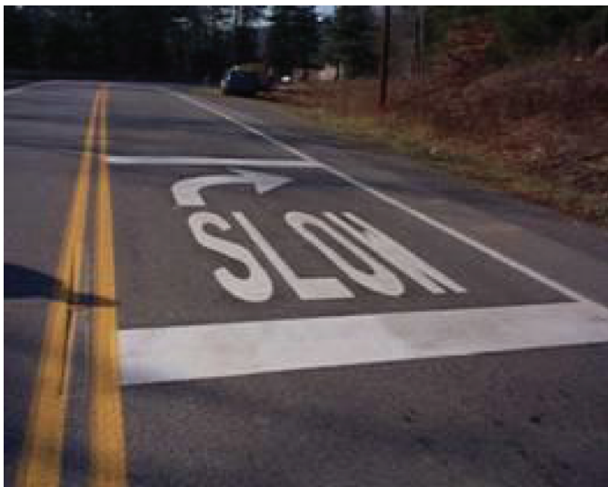
Figure 3. Example of a curve warning pavement marking (16).
