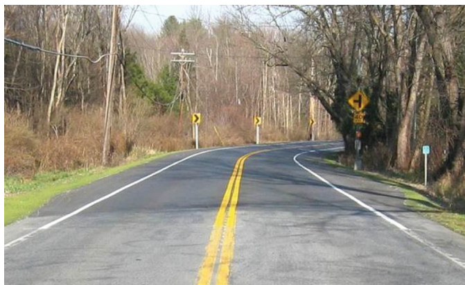
Figure 15. Shoulder widening on the inside and outside of the curve (12).
