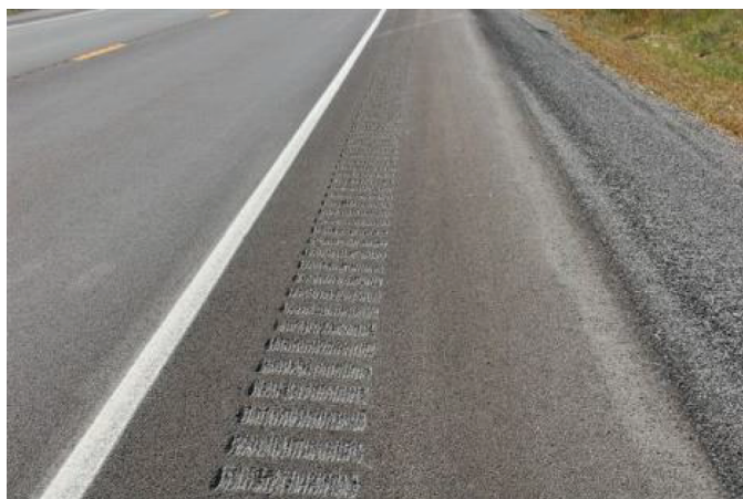
Figure 12. Example of a milled shoulder rumble stripe.
