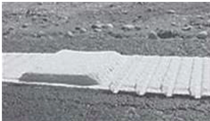
Figure 13. Example of profiled pavement marking (12).
