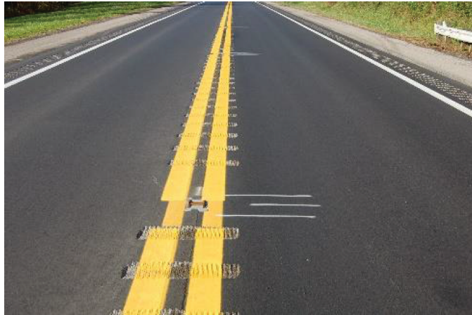
Figure 10. Example of a milled centerline rumble stripe.
