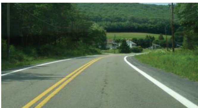
Figure 2. Roadway with 8-in. edge line (12).
