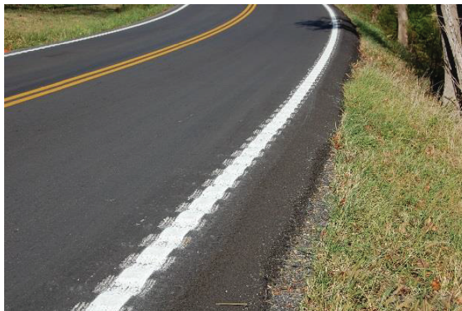
Figure 11. Example of a milled edge-line rumble stripe.
