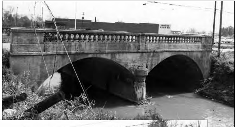
Figure IV-11, Various Decorative Treatments on Concrete Arch Bridges: Top , urn shaped balusters on the rail, (#103, 95-02036-01.51, Main Street in Watertown), built by Luten in 1921; below , modillions, incised lines in a chevron pattern, and a band along the arch; on a few bridges, this line was scored to imitate masonry, (#118, 15-SR009-21.60, built 1928, east of Newport;
