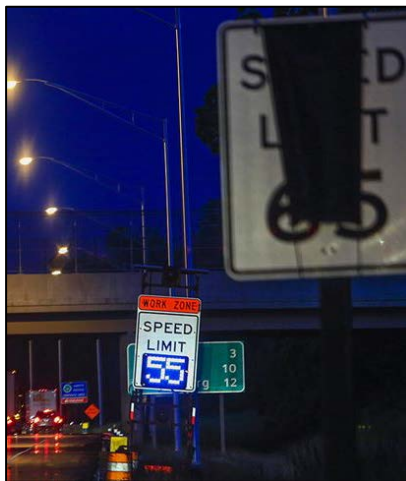
Improperly Covered Sign
