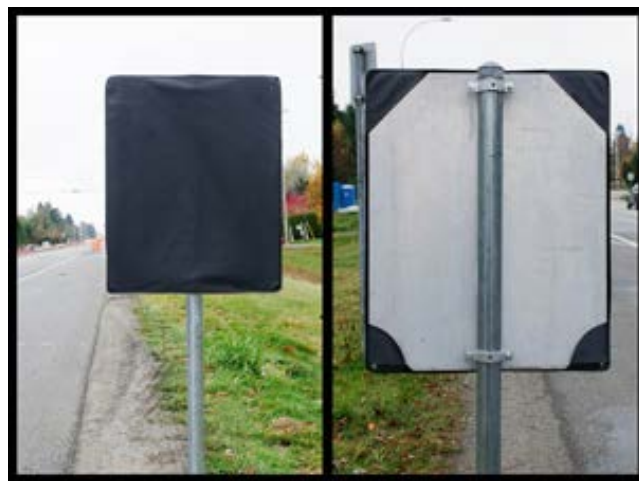
Properly Covered Sign
