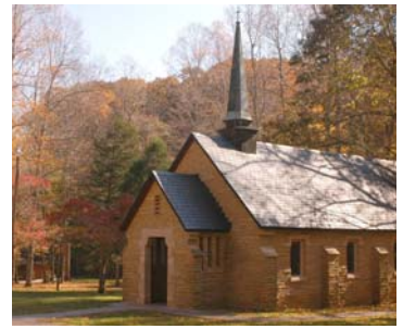
The first Cumberland Presbyterian Church at Montgomery Bell.
