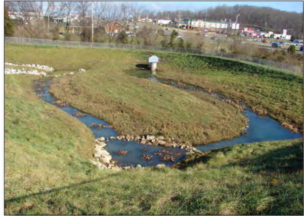
Figure 2. Partners installed a constructed urban wetland pond along College Creek.
