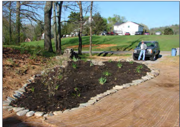
Figure 3. Partners installed a rain garden along College Creek.
