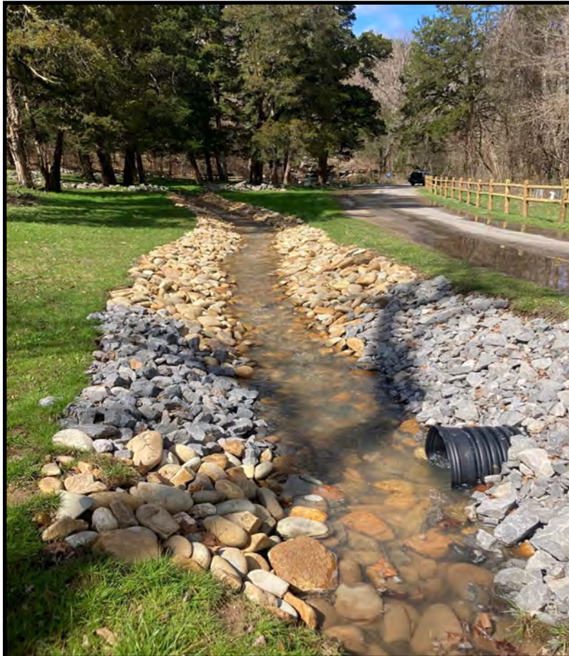
Above: Rock-lined waterway and replaced culvert at "the boils"
