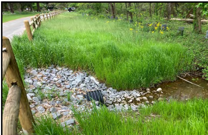
Below: Outlet of replaced culvert and view of seeded area and split rail fence
