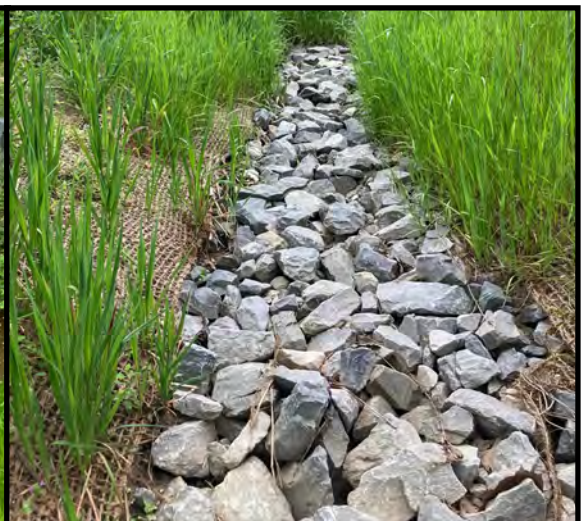
Below: Outlet of bioretention area along Valley View Highway
