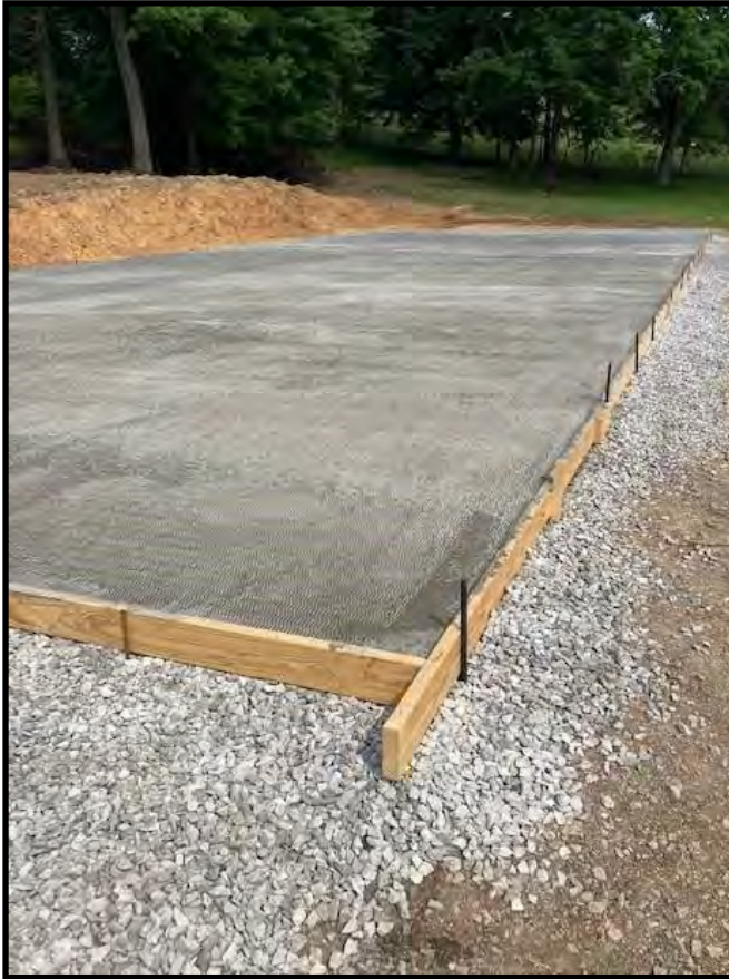
Above: 1,800 square feet heavy use area protection was installed to allow the landowner to manage his animal waste during winter feedings and prevent NPS pollutants from entering Little Sycamore Creek .
