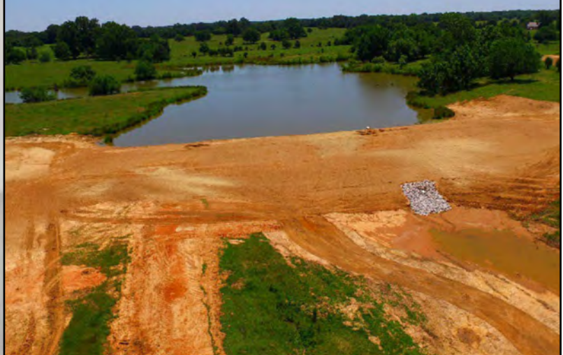
Grade stabilization structure and critical area treatment installed at Sam Pleasants Cattle Farm in Fayette County, supported by ARCF
