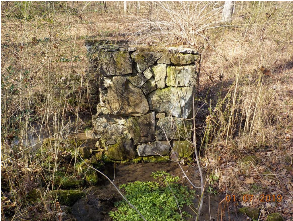
Figure 6. Springbox
